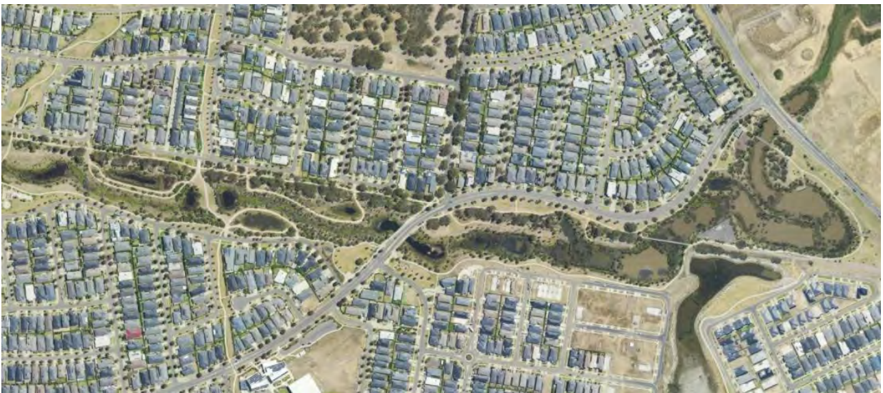
FIGURE 6-8 LINEAR WETLAND SYSTEM AT ARMSTRONG CREEK (SOURCE: METROMAP IMAGERY)
