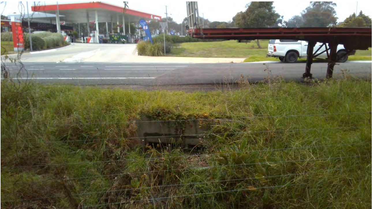
FIGURE 3-4 BYPASS BASIN OUTLET INTO THE WATERWAY AT JETTY ROAD
