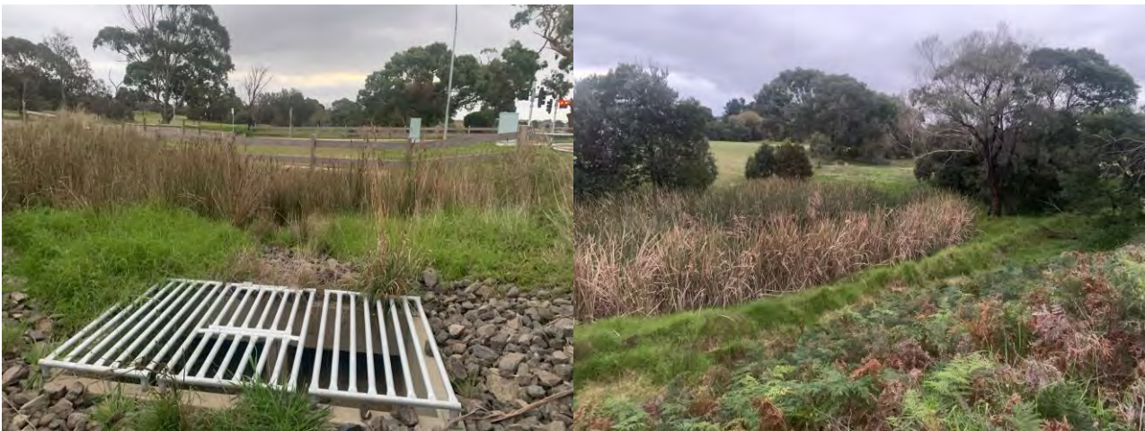
FIGURE 7-1 LEFT: GRATED PIT UPSTREAM OF TIVOLI DRIVE & RIGHT: DAM LOCATED UPSTREAM OF THE CULVERT UNDER RAIL TRAIL EMBANKMENT
