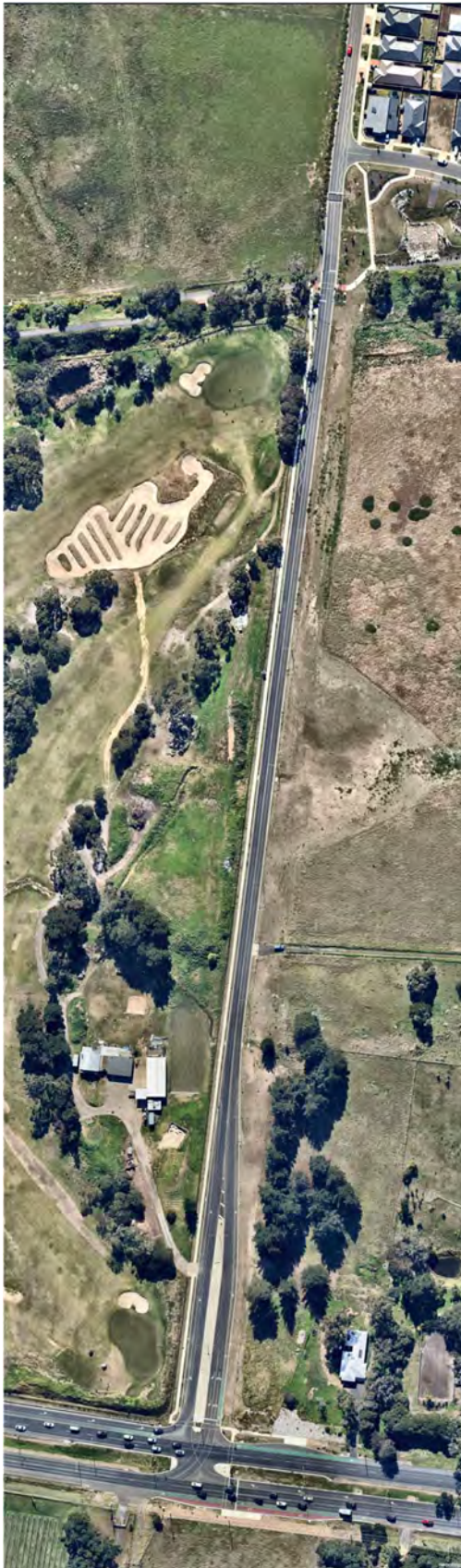
Figure 3.2: Tivoli Drive looking south near Stanley Avenue
