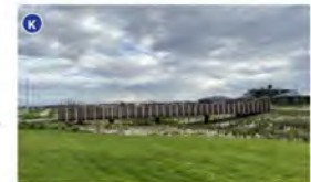
Pedestrian Bridge at The Grove Estate, Tarnet
