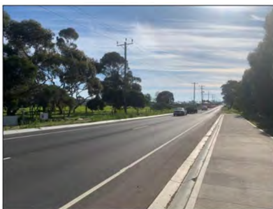
Figure 6: Jetty Road - view north
