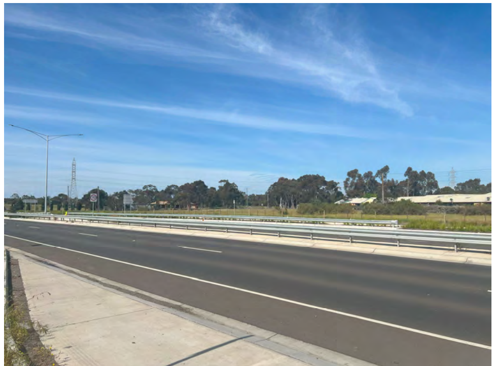
Figure 34 - Median and edge safety barriers along Barwon Heads Road (Looking south-west across the road from the bus stop, towards 25 Horseshoe Bend Road)
