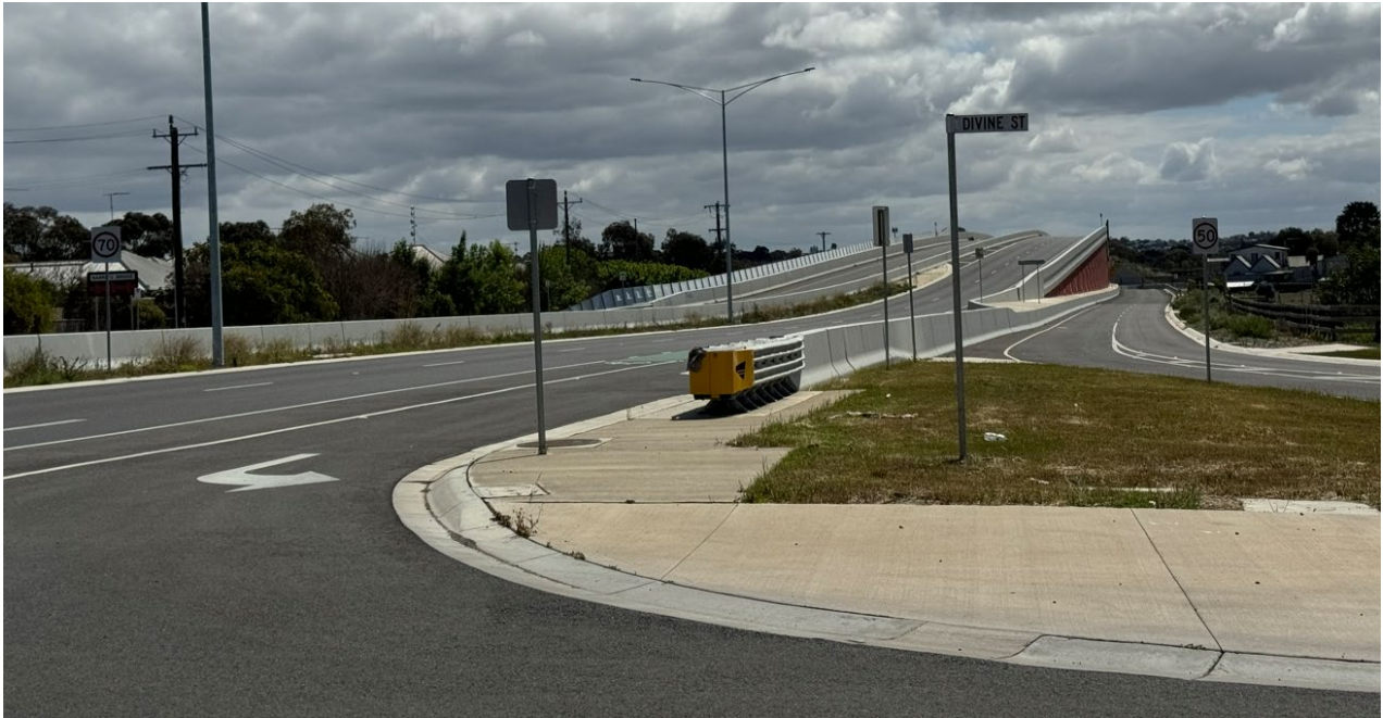
Figure 3: Photo looking north-west to the overpass from intersection of Barwon Heads Rd and Devine St
