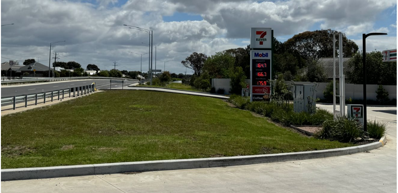
Figure 5: Photo looking north-west across frontage of Property 36
