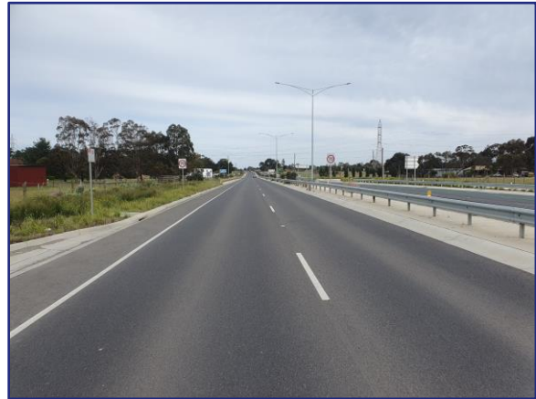
Figure 12: Barwon Heads Rd SE Bound Carriageway – View South-East
