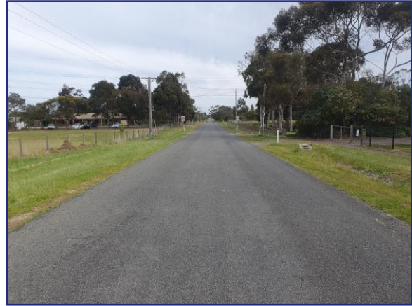
Figure 16: Horseshoe Bend Rd - View South
