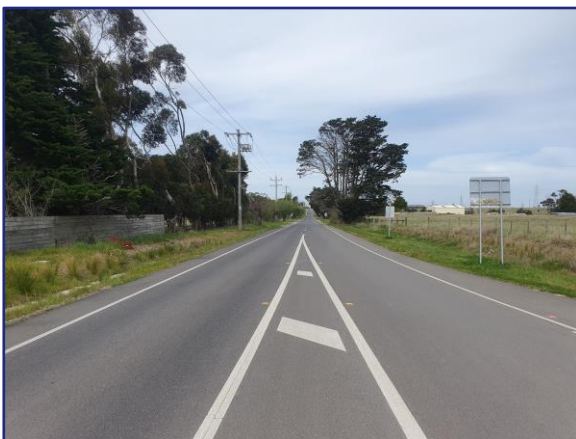
Figure 13: Tannery Rd - View East
