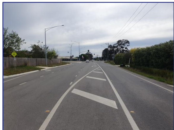
Figure 14: Tannery Rd - View West
