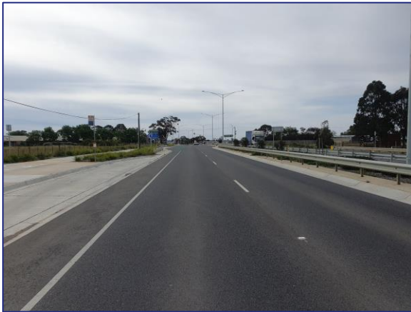
Figure 9: Barwon Heads Rd NW Bound Carriageway – View North-West
