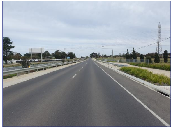
Figure 10: Barwon Heads Rd NW Bound Carriageway – View South-East
