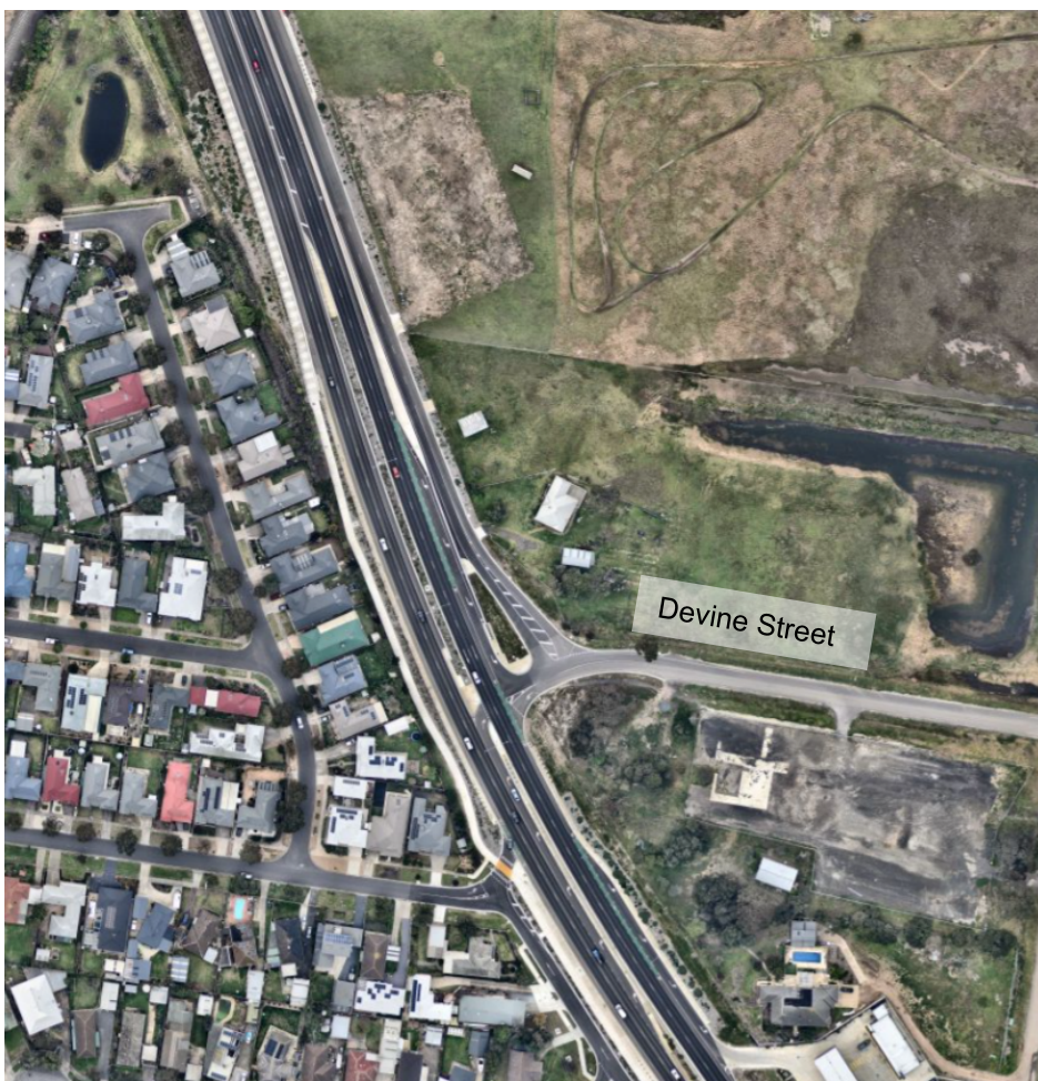
Figure 6.3: Barwon Heads Road / Devine Street intersection (reproduced with permission from Nearmap)
