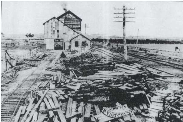
Pipe factory under construction, 1912. Source: News of the Week , 22 August 1912, p.15.
