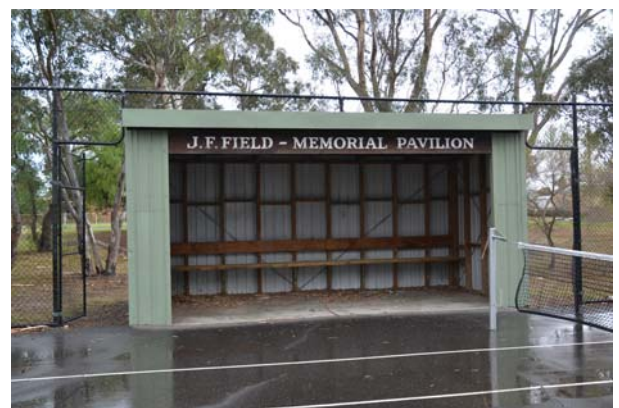
J.F. Field Memorial Tennis Pavilion, east elevation.
