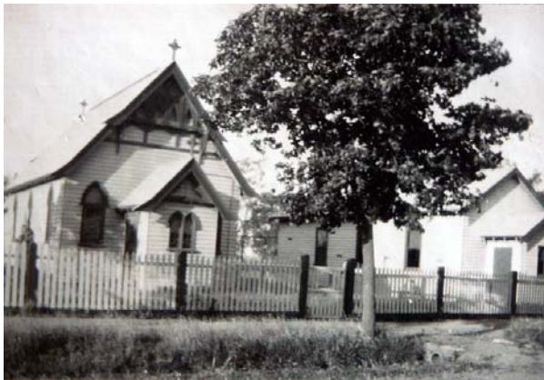
St. Cuthbert's Church (left) & Hall (right) fronting Marshalltown Road, c.1928. Source: Holmes collection c/o David Rowe.
