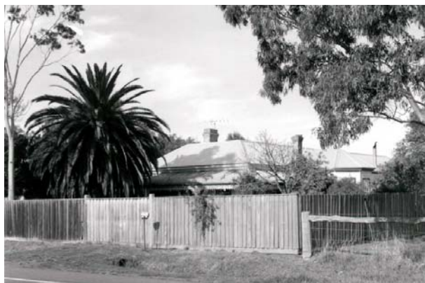
28 Marshalltown Road, 19 May 1998. Source: D. Rowe & L. Huddle, 'Outer Areas Heritage Study Stage 2'.
