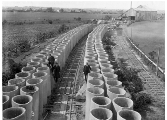
Curing yard showing recently manufactured pipes, c.1913. Source: Barwon Water archives.
