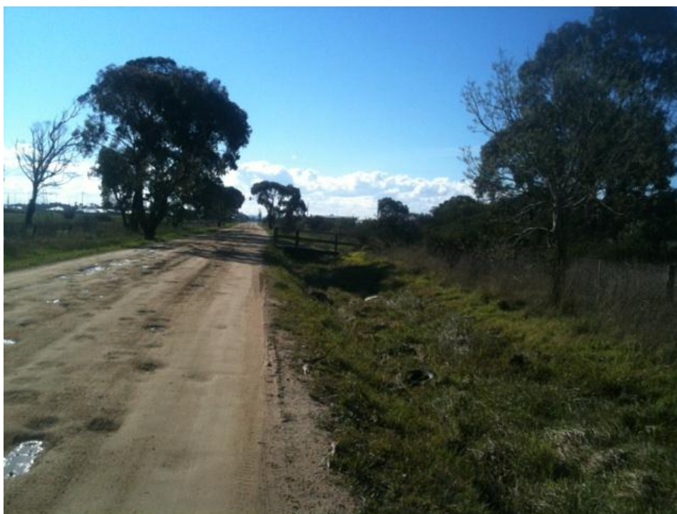
Plate 2: Drews Road looking north, showing drainage ditch.
