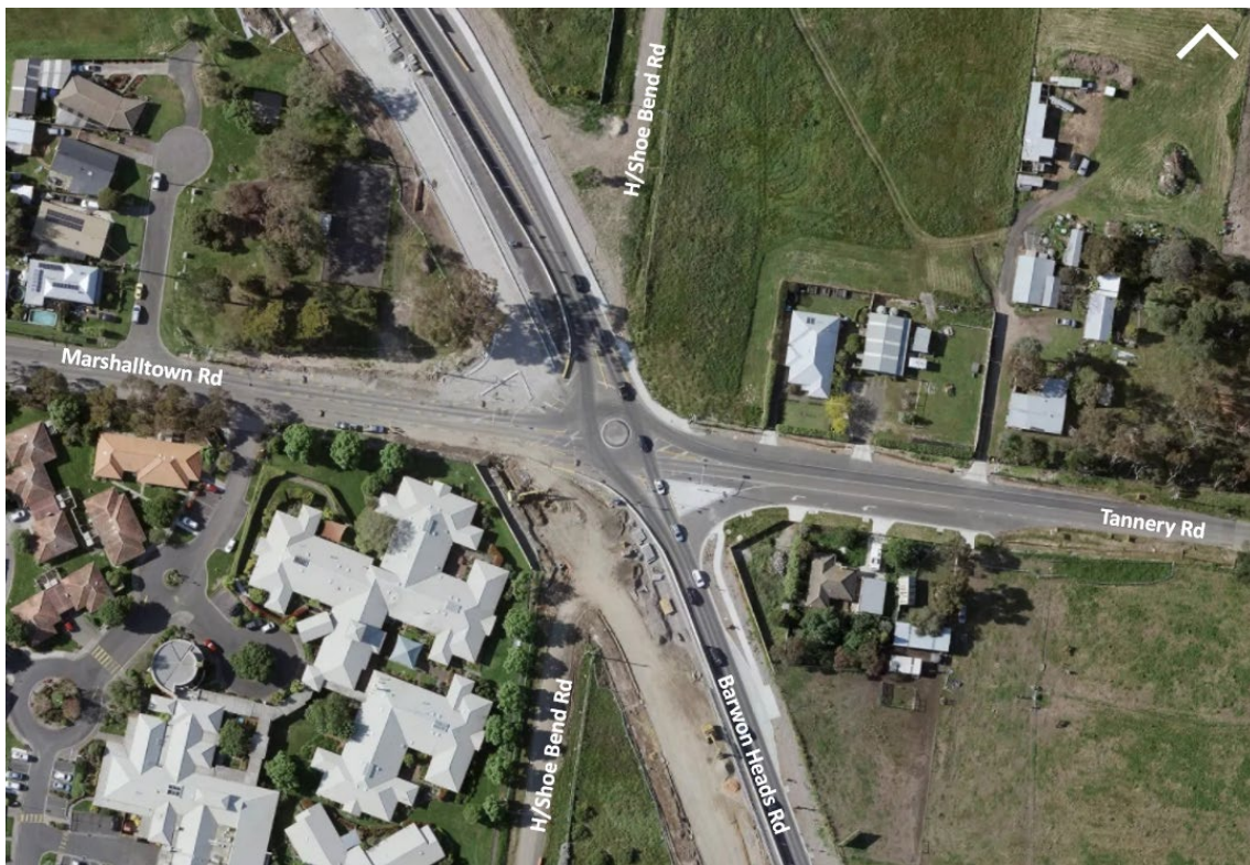
Figure 2-5: Barwon Heads Road/Marshalltown Road Intersection (Under Construction)
