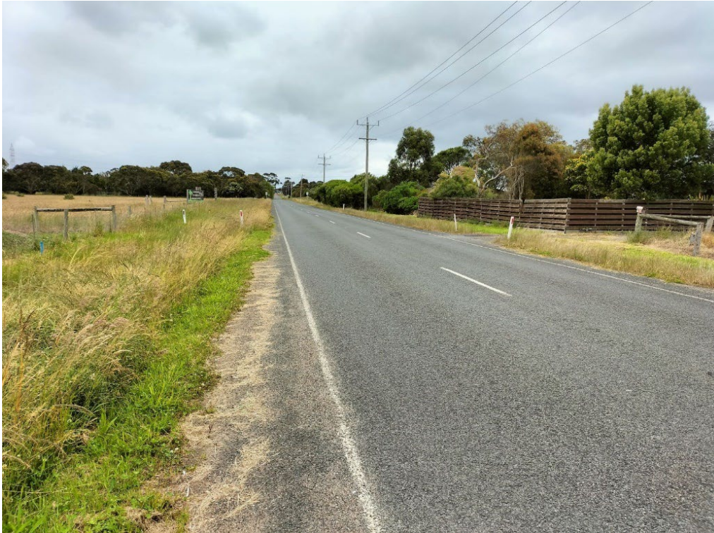
Figure 2-14: Horseshoe Bend Road looking north, from north of Reserve Road
