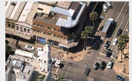
Image above: Electronic signage as constructed at 165 Moorabool Street, Geelong (Nearmap, 25 November 2020)
