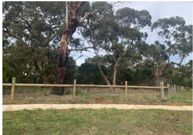
Fencing adjoining Yellow Gum Bushland Reserve
