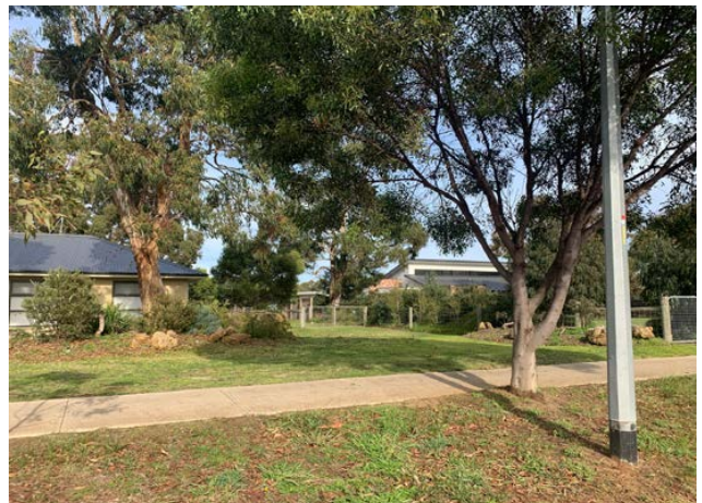
Post and wire side fence with partial timber paling
