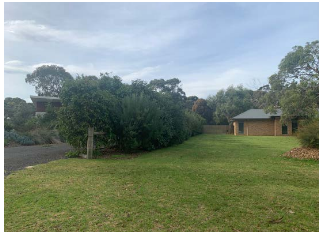
Timber paling fence providing security to rear garden
