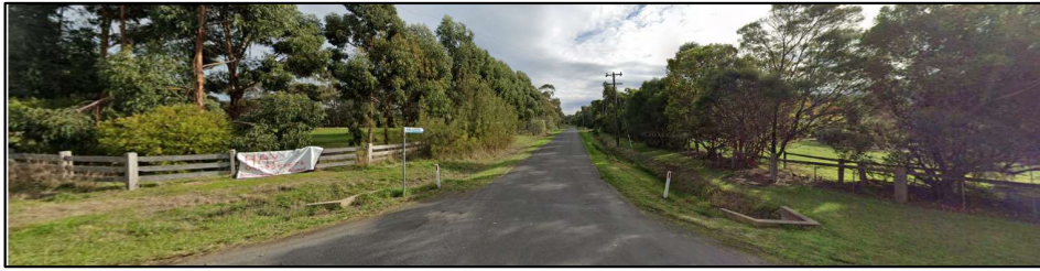
Figure 29 - View west down Kalkarra Drv at the Horseshoe Bend intersection (pink arrow) with LDRZ subdivision to the left and right. Source: Google street view
