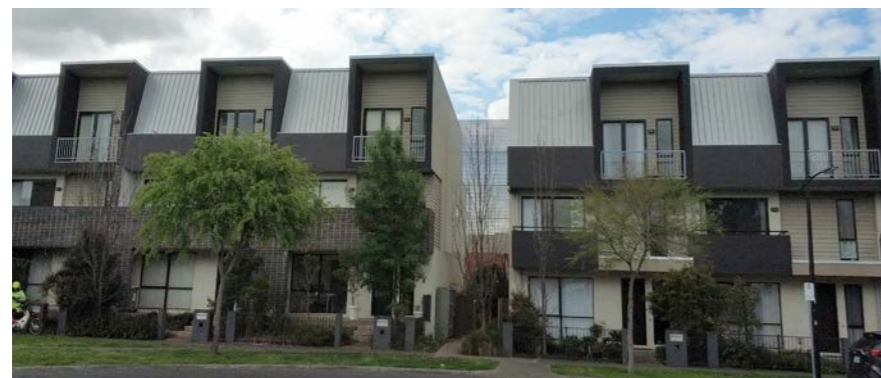
3 STOREY ROW HOUSE WITH NO REAR COURTYARD
