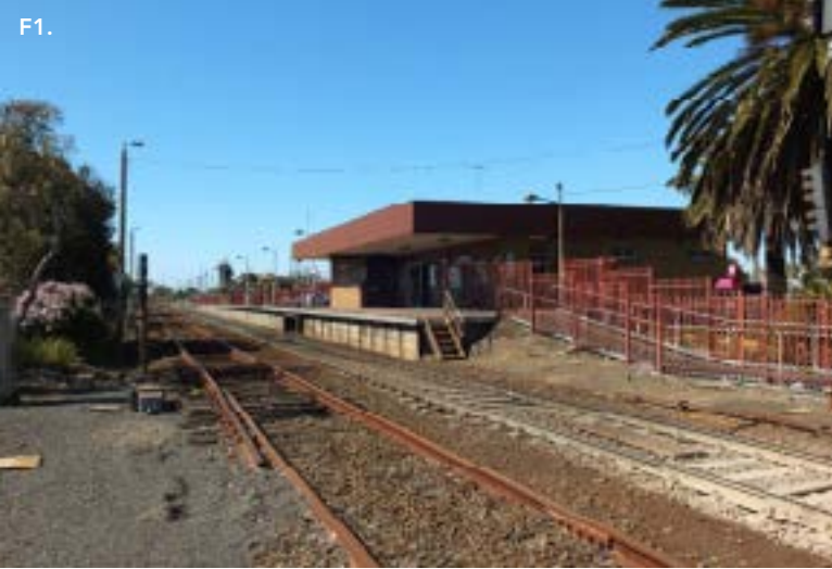
The central core of the study area is the South Geelong Railway Station site. It is defined by a single storey, flat-roofed brick station building (Figure 1) constructed in 1984 immediately south of the railway lines, towards the west end. Much of the site is taken up by sealed car parking. Near the west boundary are three mature Canary Island Date Palm trees.
