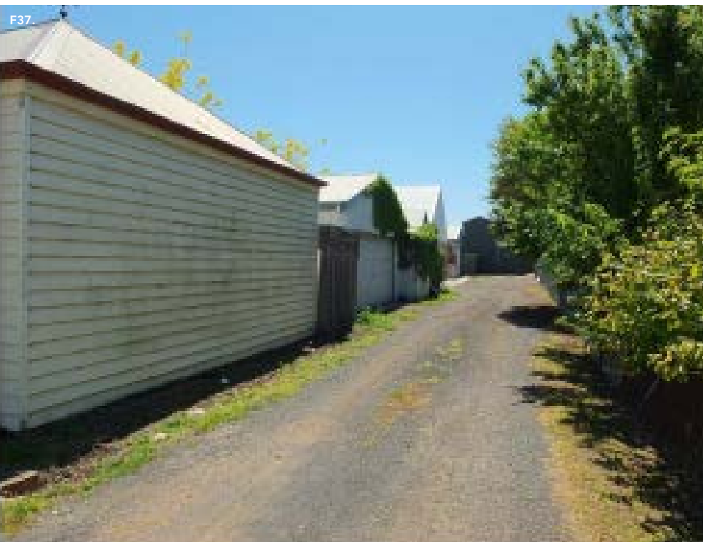
Figure 37. Garaging fronting rear lane off Richmond Place, 2019.
