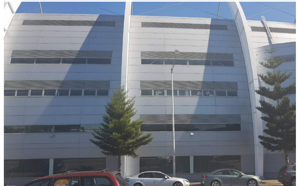
Figure 78. Existing conditions along Moorabool Street
