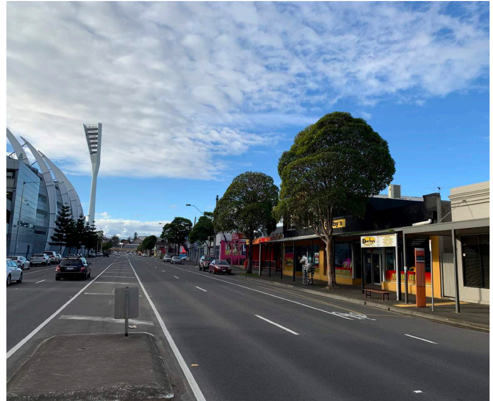
Figure 77. Existing conditions along Moorabool Street
