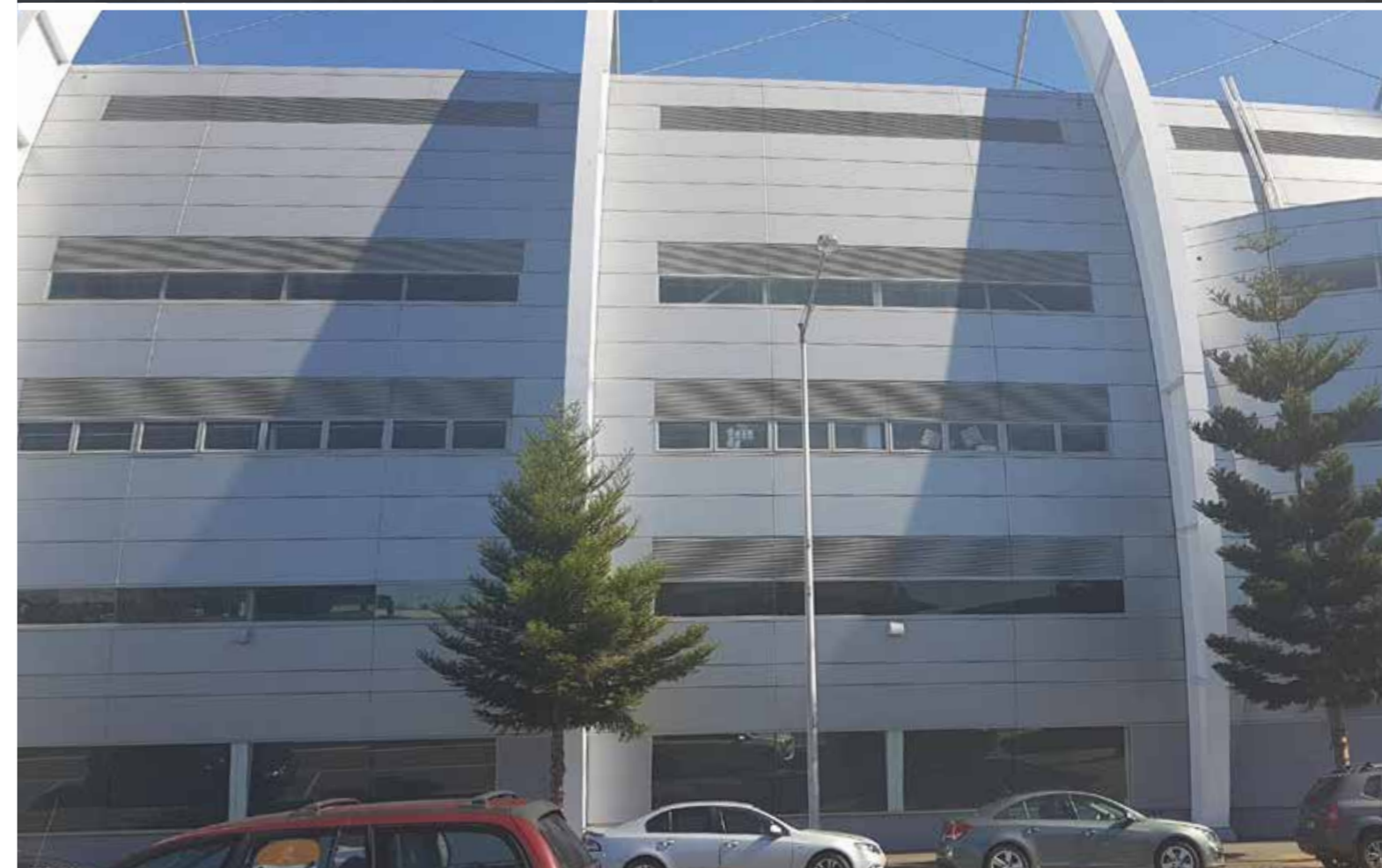
Figure 78. Existing conditions along Moorabool Street
