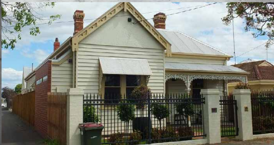
Figure 7: House, Barwon Terrace (between Moorabool & Yarra Streets), n.d., occupied by Edward Willis in the 1840s (and owned by David Fisher). Source: Ian Wynd collection, Authentic Heritage Services
