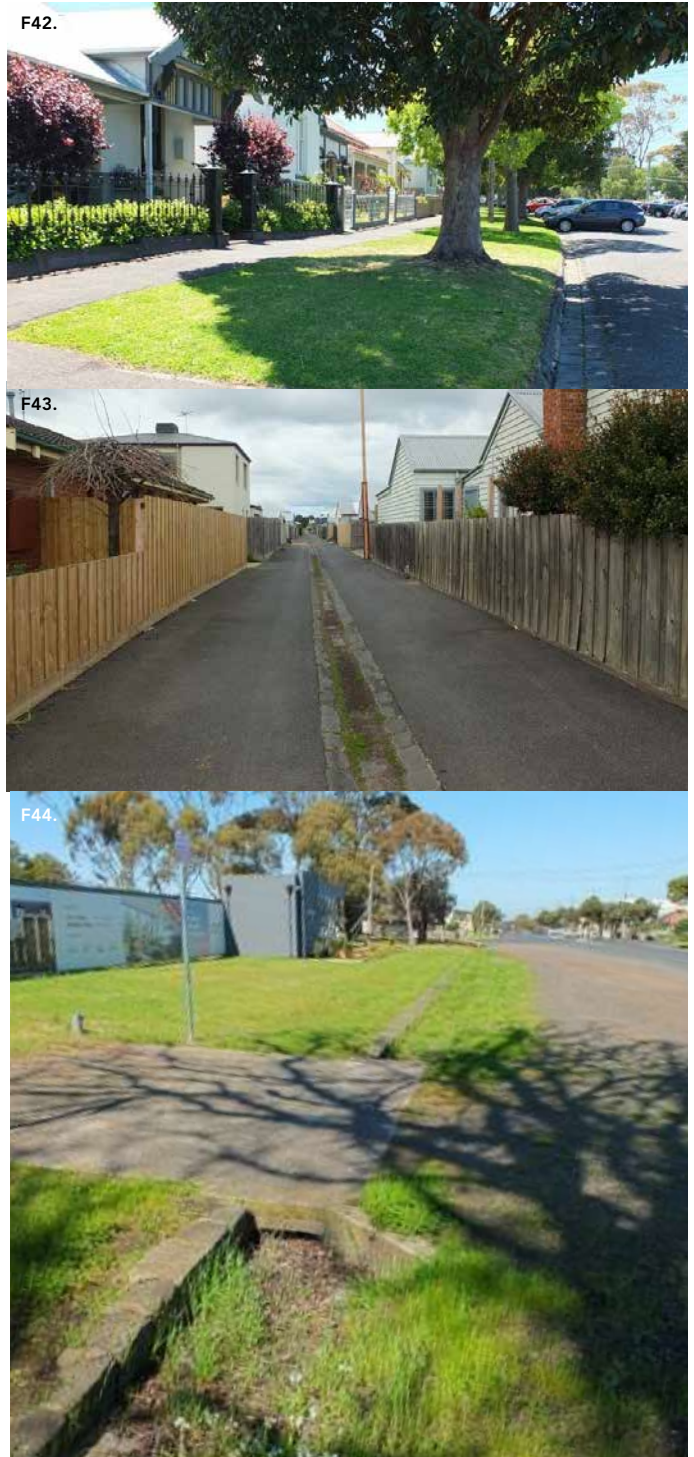
Figure 42. Asphalt footpaths and early bluestone kerb and channel, Bourke Crescent, 2019.
