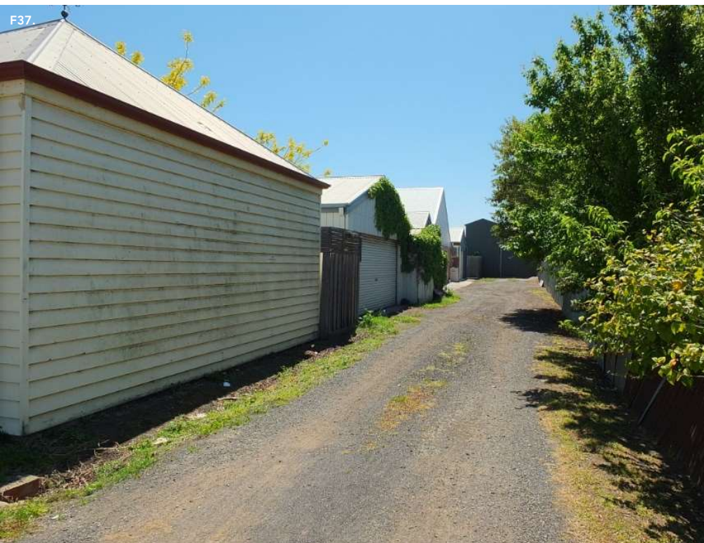
Figure 37. Garaging fronting rear lane off Richmond Place, 2019.
