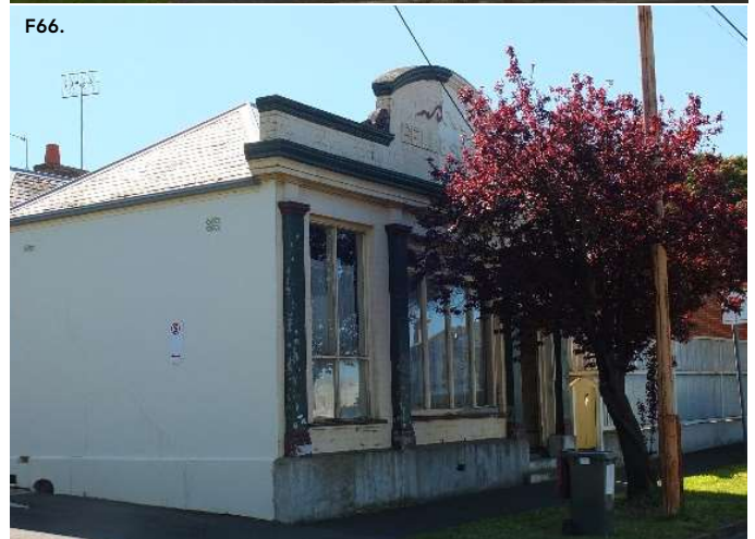
Figure 65. Former candle factory, 80 McKillop Street, 2019.
