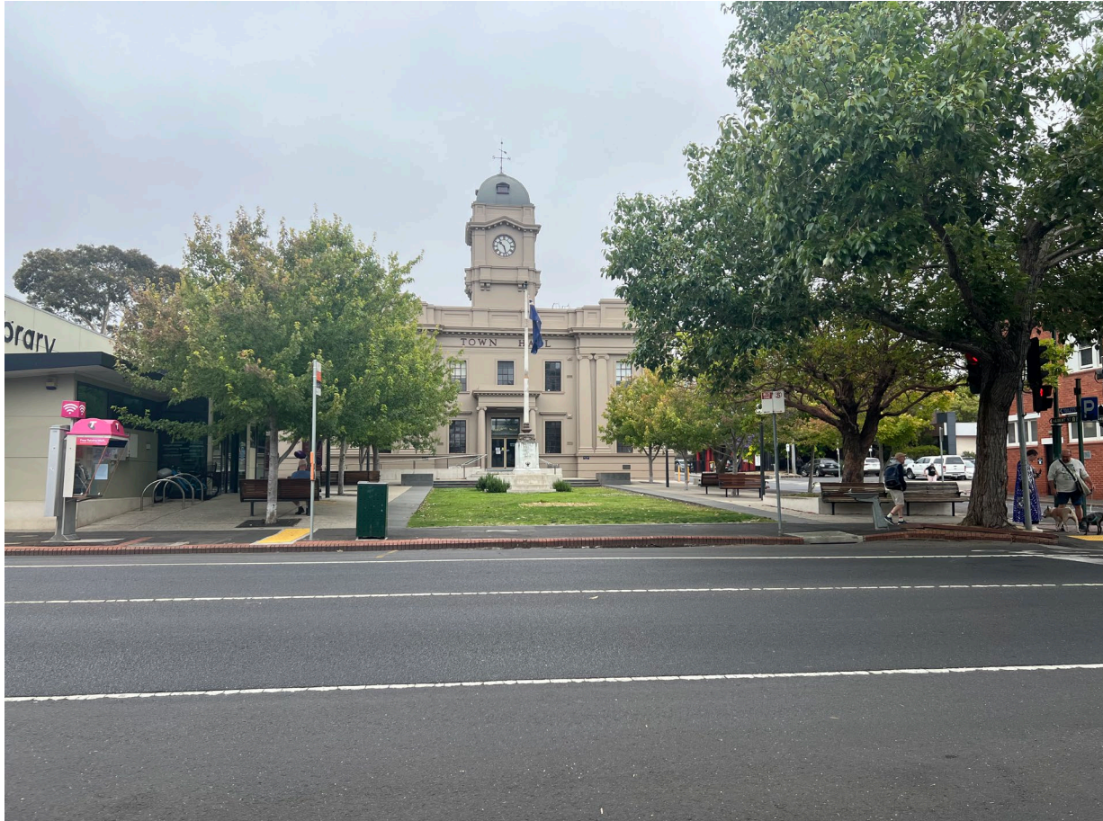
Town Hall building (corner Pakington Street and Albert Street)
