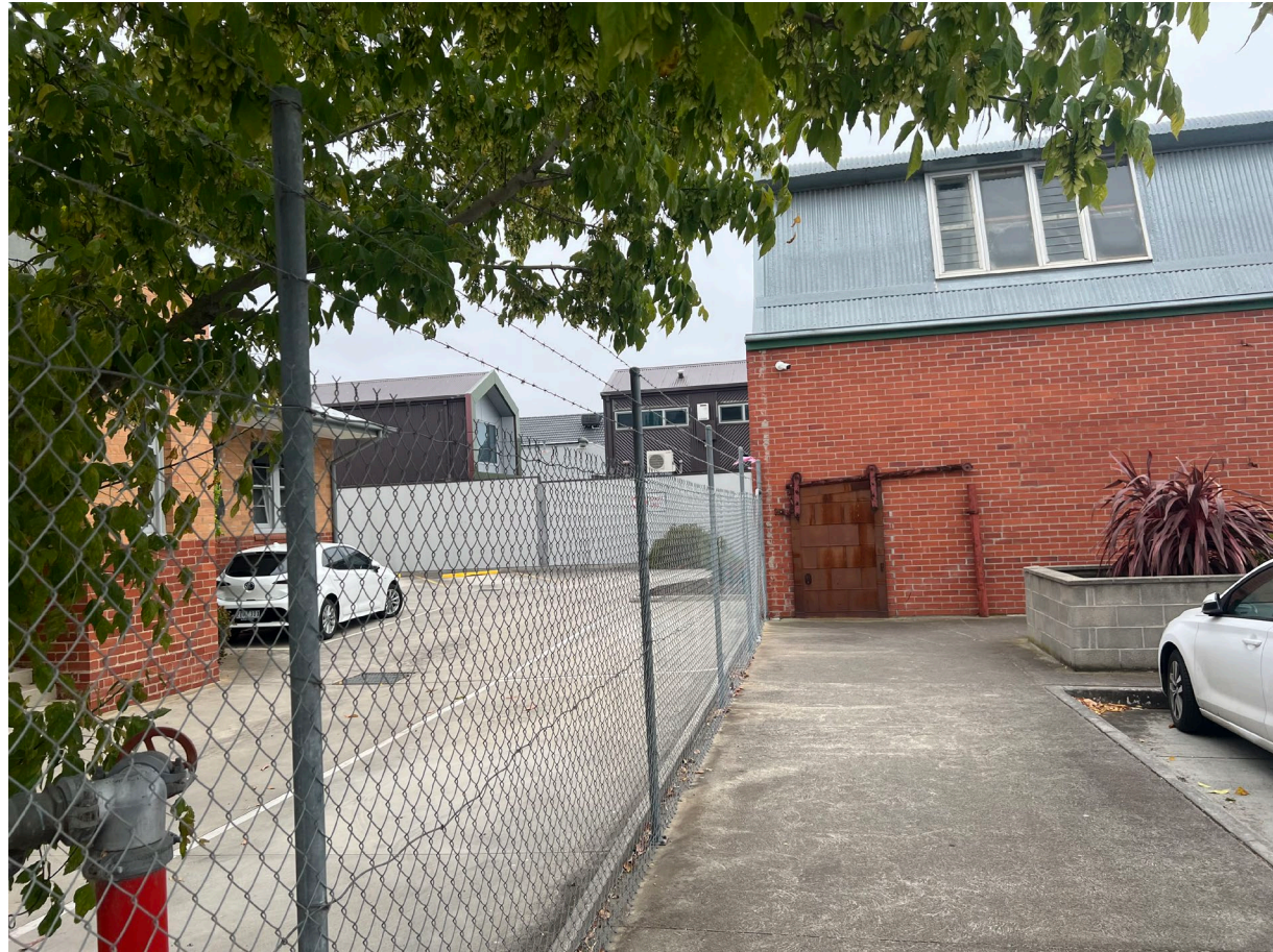
Former Donaghy's Walk Building
