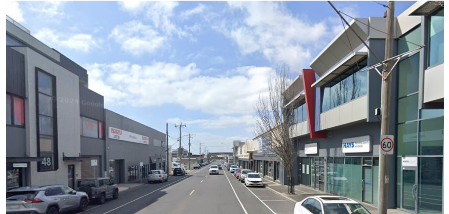
Figure 04: Gordon Ave, looking east towards Geelong CBD (Google maps, 2025)
