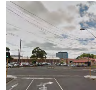
Latrobe Terrace and Gordon Avenue intersection.
