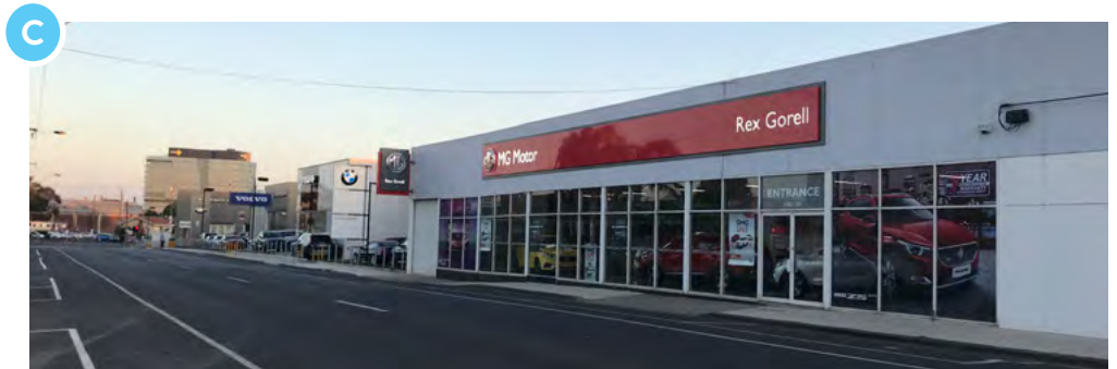
Existing car dealerships in large buildings with wide frontages along Gordon Avenue.
