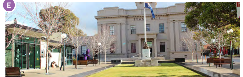
Geelong West library and Town Hall along Pakington Street near corner of Albert Street.
