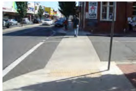
Northcote Raised Threshold Treatment, City of Darebin
