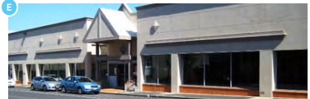
Large building with wide frontage along Gordon Avenue.
