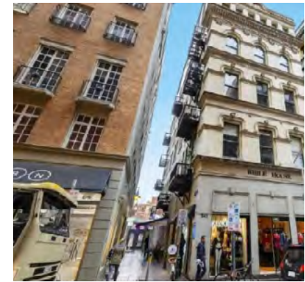
Scott Alley in Melbourne demonstrates that this scale of built form can be supported along a narrow laneway due to the short length of the laneway.
