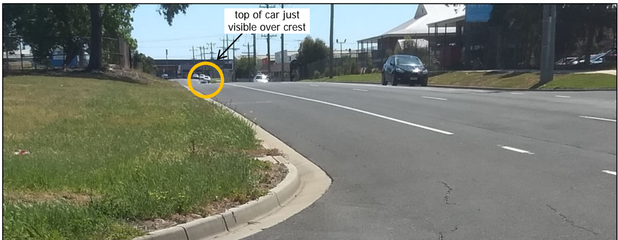
Figure 5.13 View North along Weddell Road from Existing Saleyards Access
