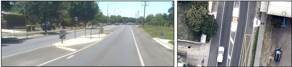
Figure 5.5 Example of Central Island Pedestrian Refuge
