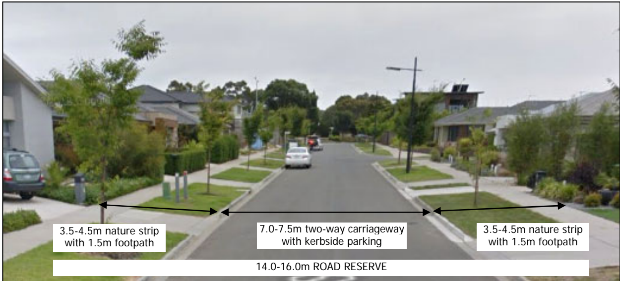
Figure 5.1 Example of a Residential Access Road
