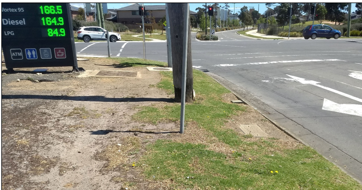
Figure 5.7 No Footpath Along Victoria Street (South Side)
