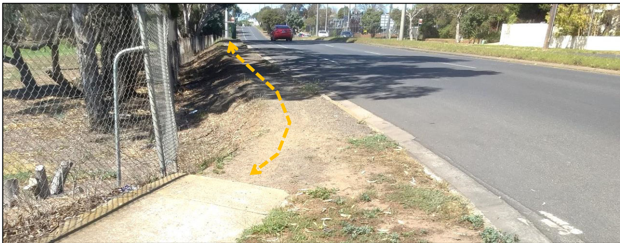
Figure 5.6 Footpath Ends 60m Short of the Bus Stop on Ballarat Road (Southeast of Thompson Road)
