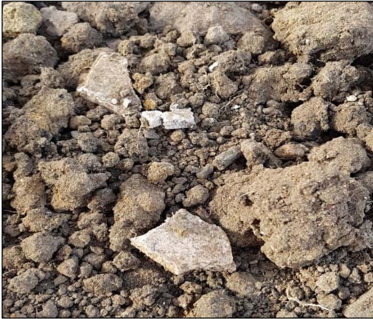
Plate 3: TP11 x4 pieces of ACM
