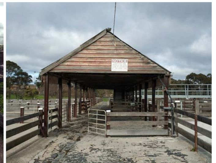
B Structure to be retained and restored for use as a picnic shelter.
