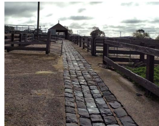
A Bluestone channel to be retained and incorporated in park design.
