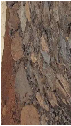
EXAMPLE OF WELL INTERLOCKED ROCKWORK WITH SEALED VOIDS
