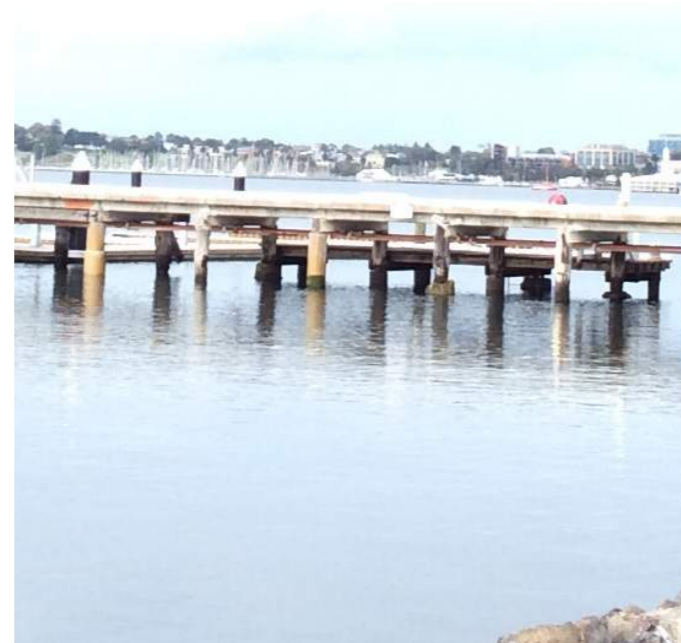
Existing pier and columns
