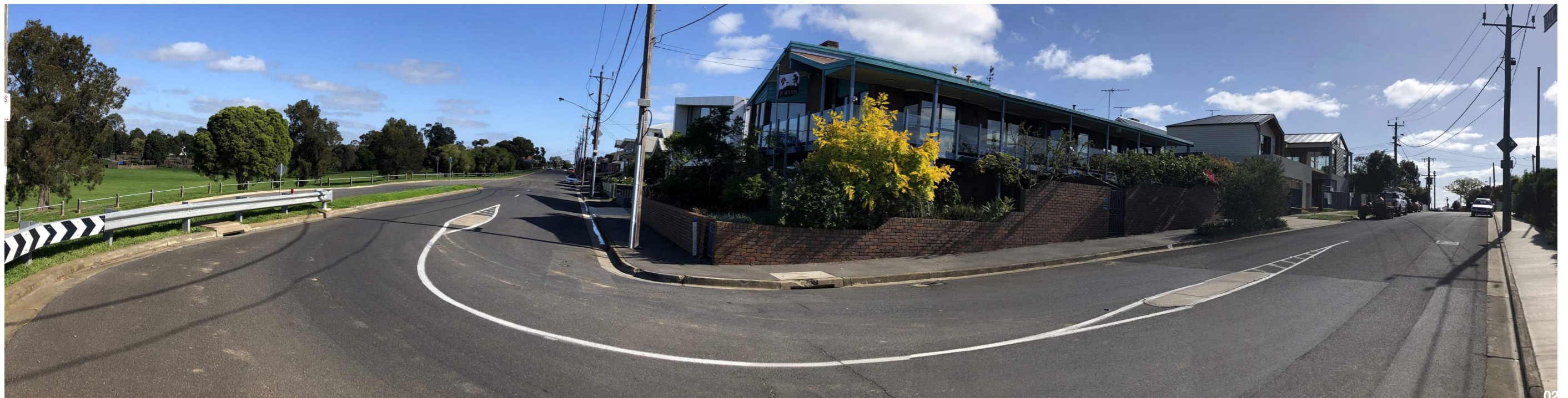
Balmoral Crescent - Looking Away From Site Down Liverpool Street
