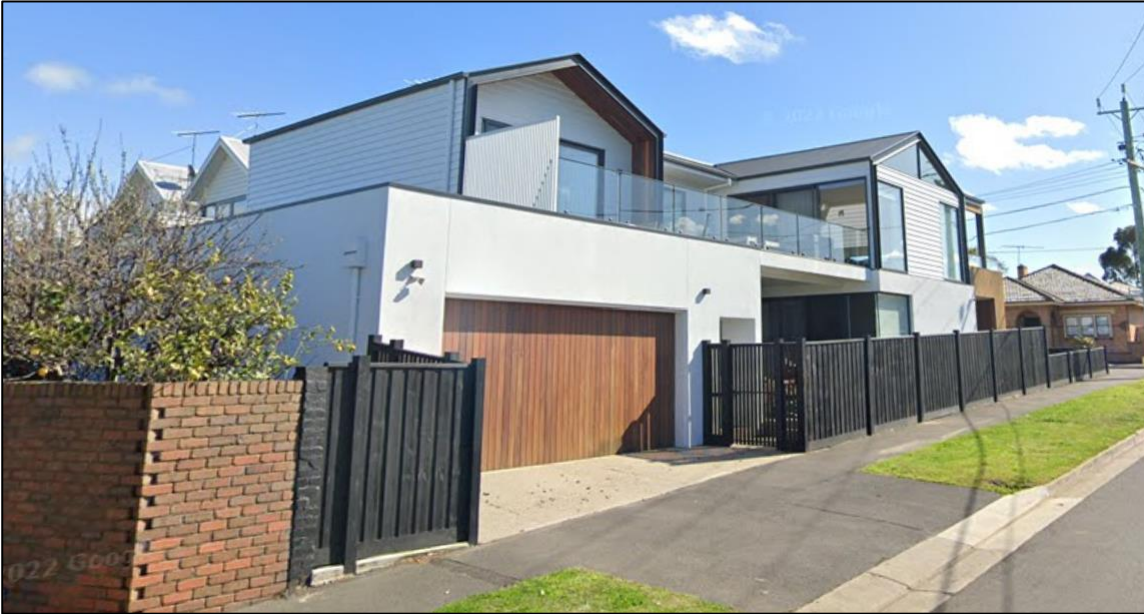
Figure 13 - View to Eastern side of 52 Walker Street taken from Balmoral Crescent adjacent to Stage 5 area
