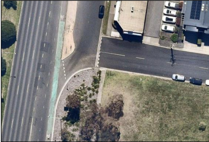
Figure 3 - Liverpool Street/ Melbourne Road intersection 6 October 2023
