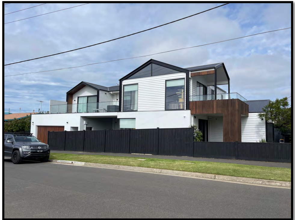
Figure 3 - 52 Walker Street, recently refurbished and extended
