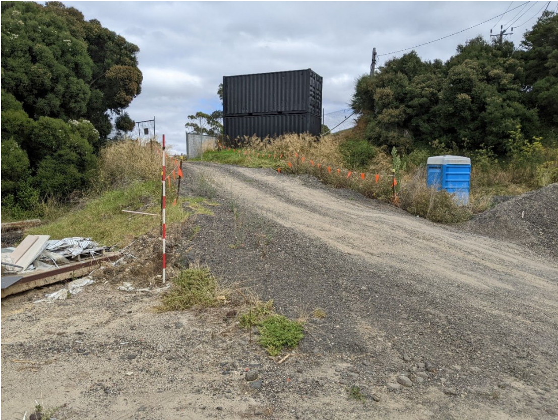
Figure 34: Gravel hard stand access ramp, facing southwest (C. Hawker, 22 February 2022)
