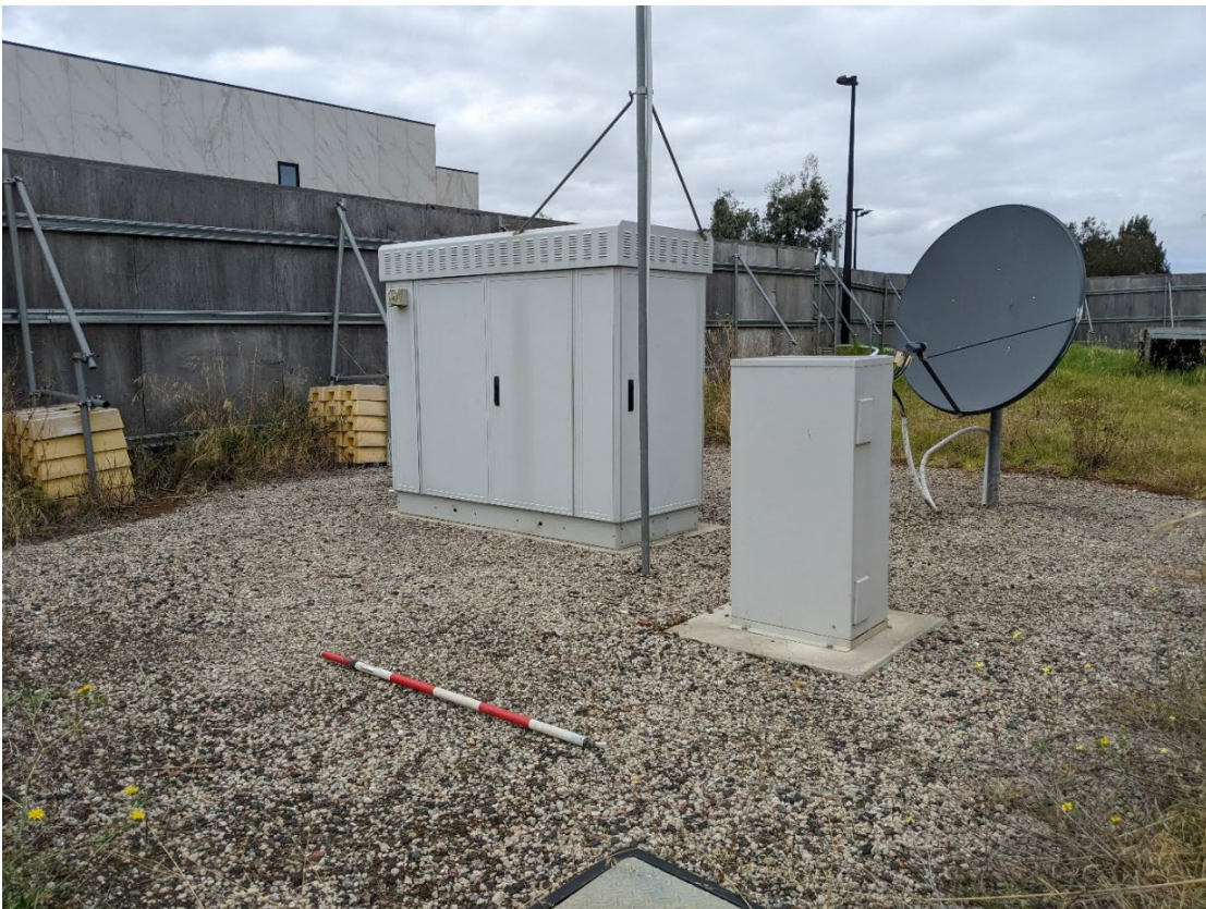
Figure 35: Installed utilities, facing southeast (C. Hawker, 22 February 2022)
