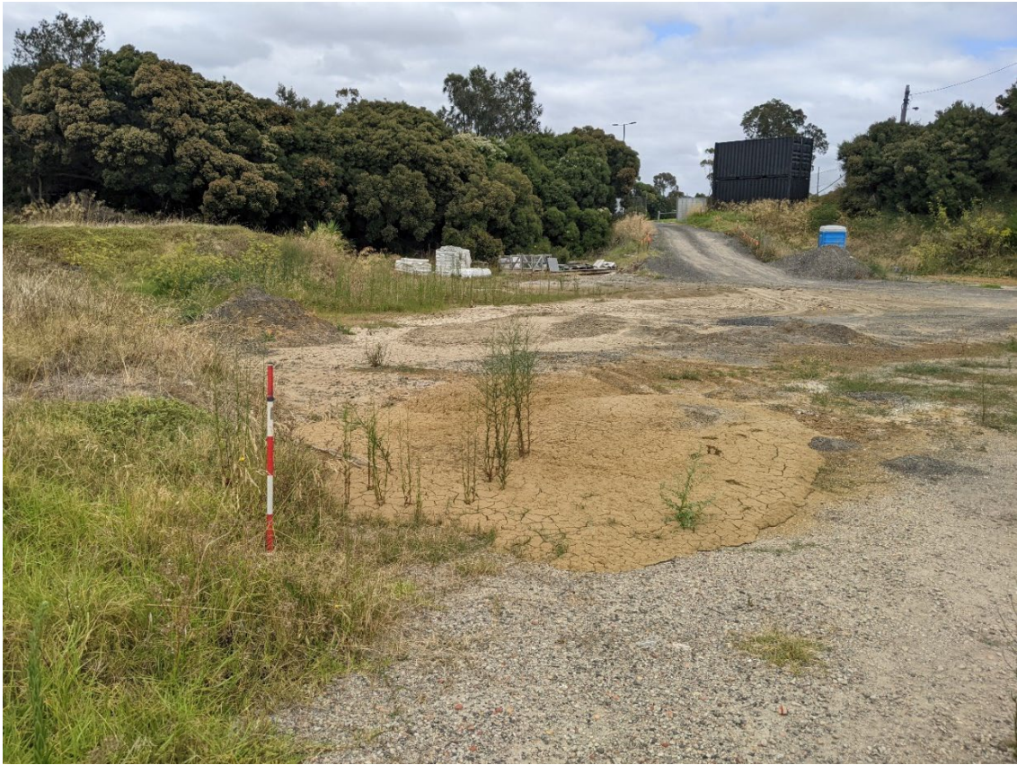
Figure 32: Gravel area and soil stockpiling, facing west (C. Hawker, 22 February 2022)
