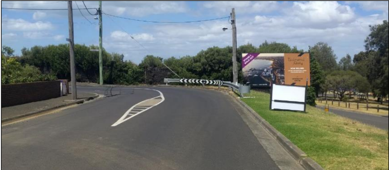
Figure 2-6 Liverpool Street (Eastbound)
