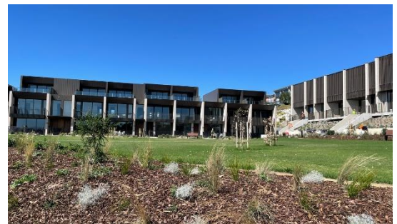
North-East – Townhouses fronting Corio Bay forming part of the Balmoral Quay development
