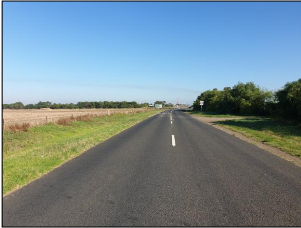
Figure 9: Canterbury Rd East - view west (east of rail line)
