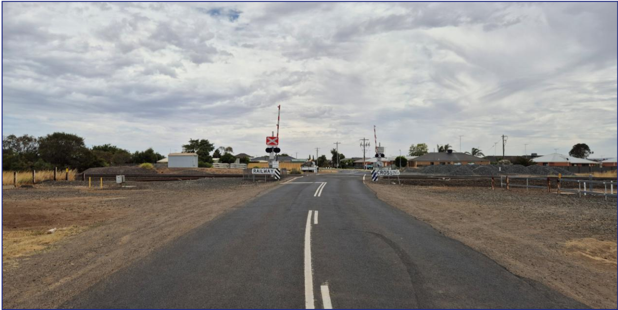
Figure 42: Level Crossing at Canterbury Road East, view west
