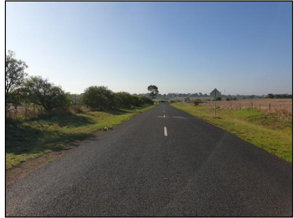
Figure 10: Canterbury Rd East - view east (east of rail line)
