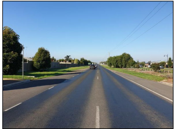
Figure 22: Forest Road South – view south from (south of Canterbury Road East)
