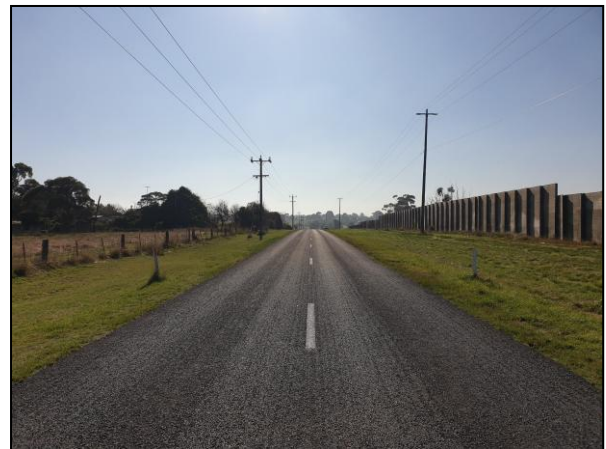
Figure 14: Rennie Street - view north-east (at subject site)
