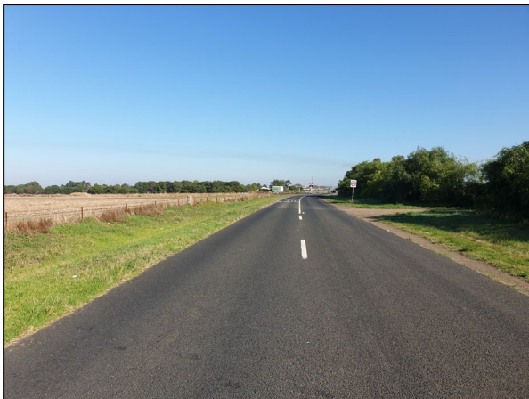
Figure 8: Canterbury Rd East - view west (east of rail line)
