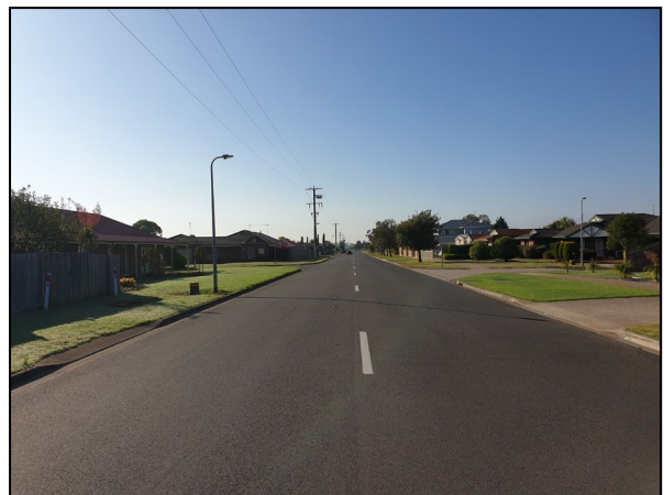
Figure 11: Canterbury Rd East - view east (west of rail line)
