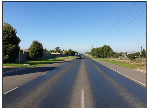
Figure 21: Forest Road South – view south from (south of Canterbury Road East)
