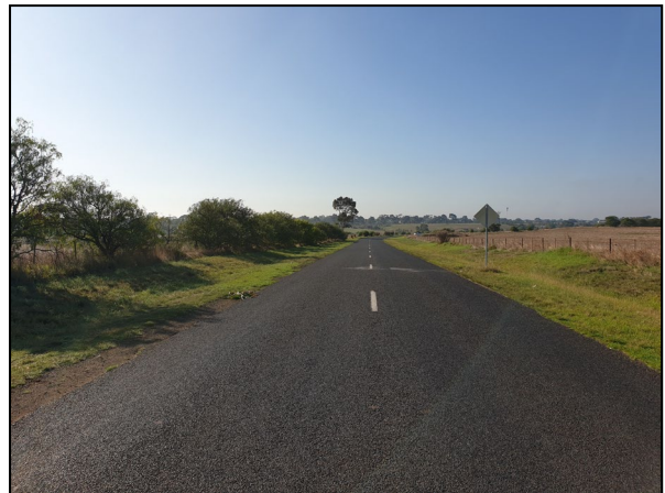
Figure 9: Canterbury Rd East - view east (east of rail line)
