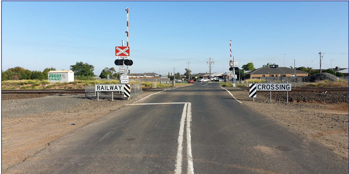
Figure 37: Level Crossing at Canterbury Road East, view west
