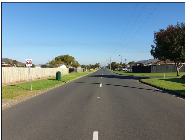
Figure 10: Canterbury Rd East - view west (west of rail line)
