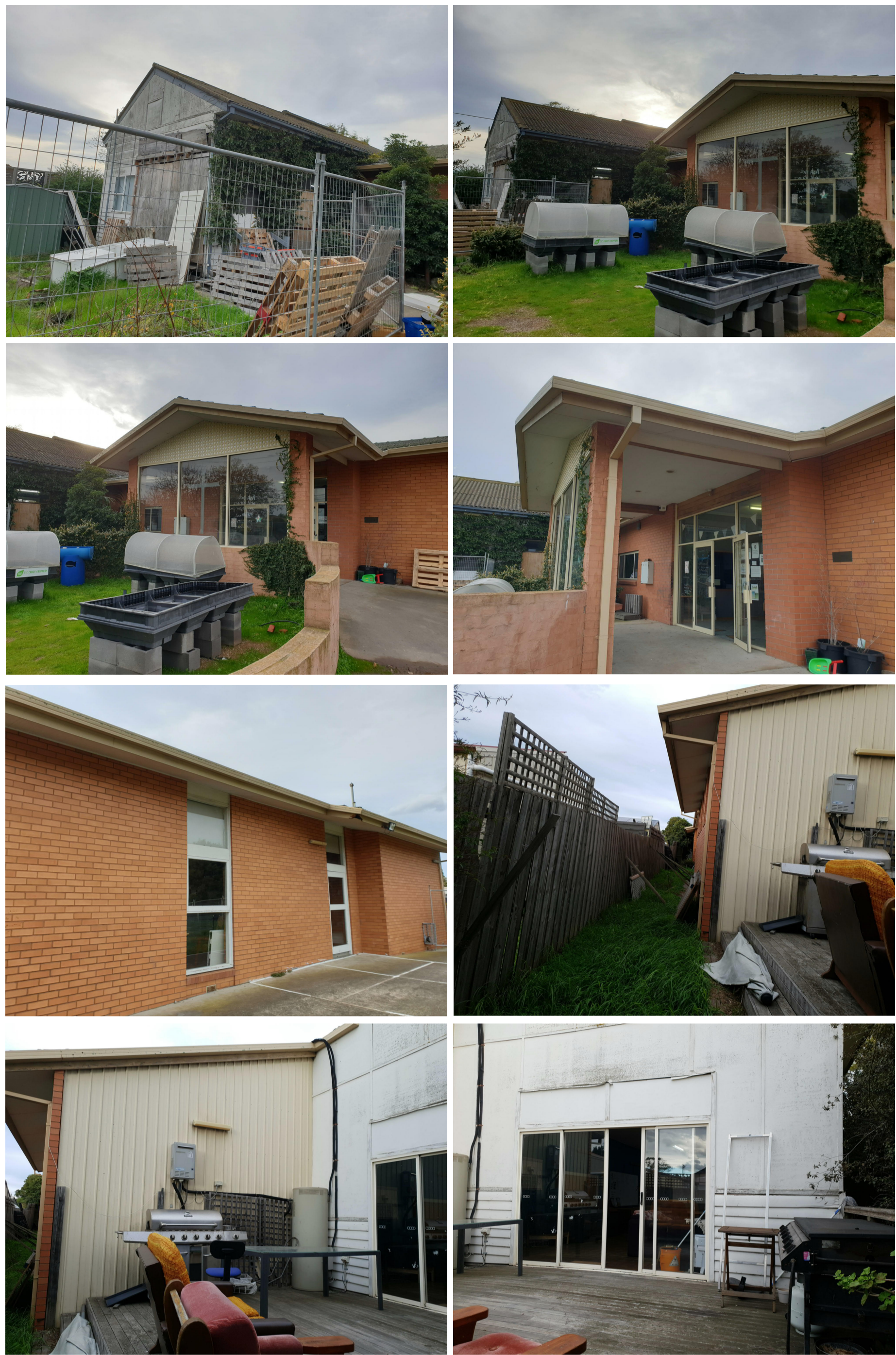
EXISTING SITE CONDITIONS PHOTOS
