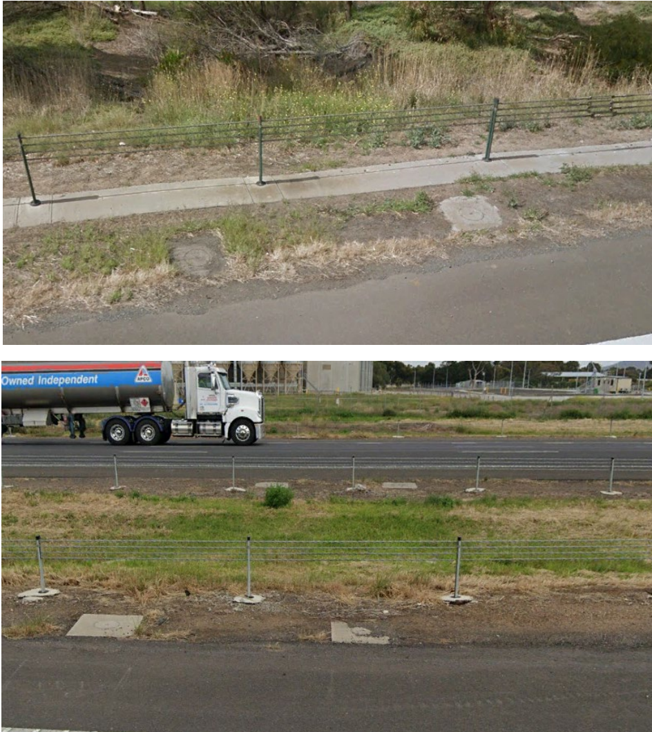
Figure 28 Princess Highway at culvert location showing side by side inspection pits
