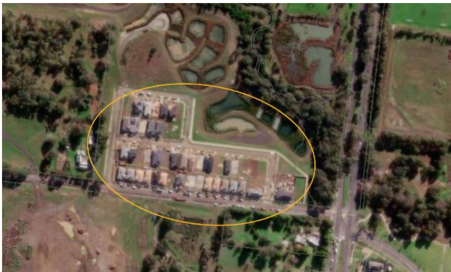
Figure 10 Recent works at Rowands Street area, Armstrong Creek
