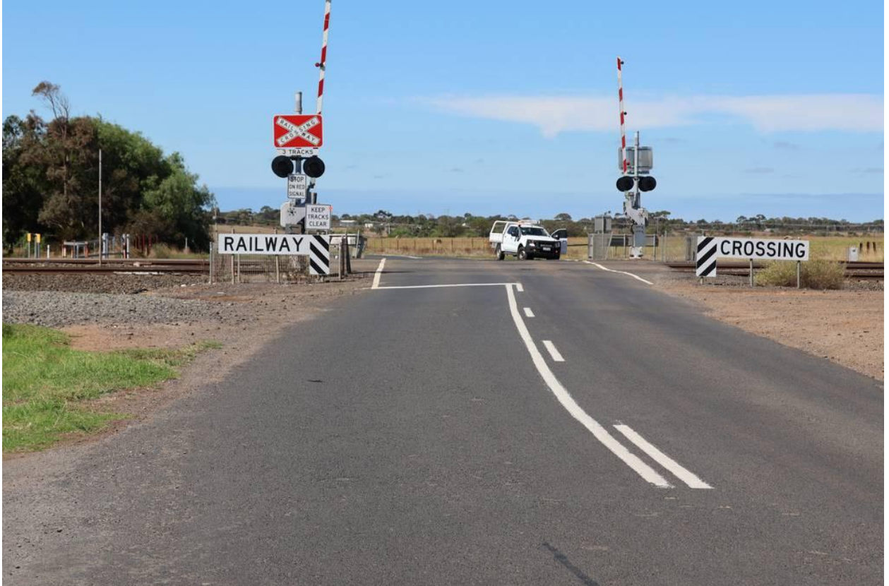
Figure 7 East bound crossing approach
