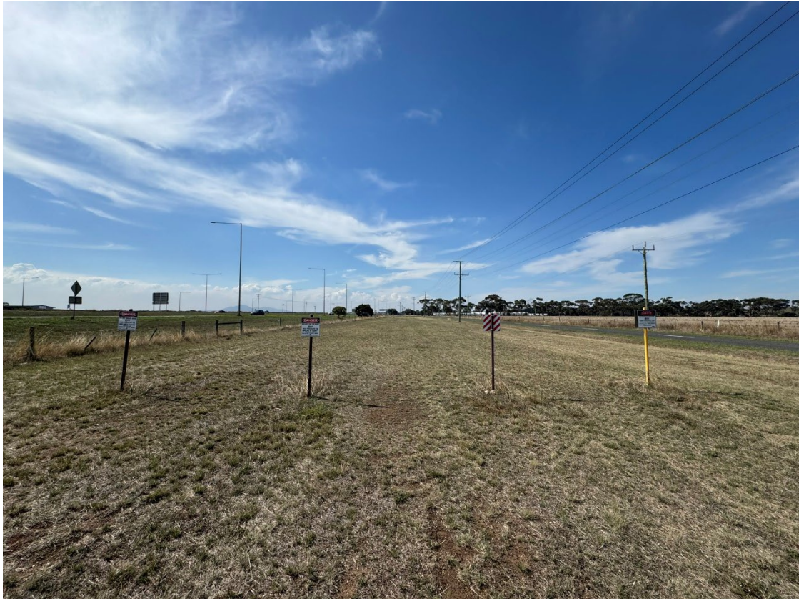
Figure 7: 1. WOPL, BOPL, WAG, and Brooklyn - Corio pipelines running in parallel (looking north east)
