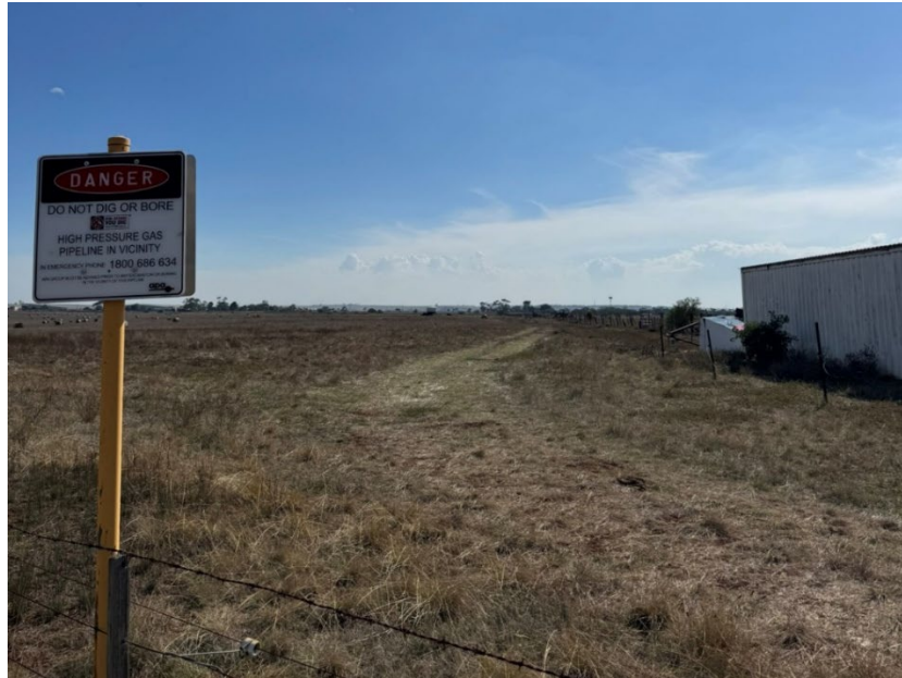
Figure 9: 3. Lara - Iona pipeline after leaving the city gate (looking west)
