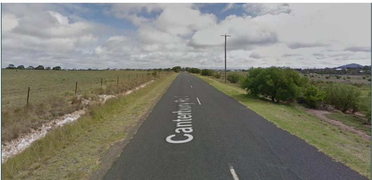
Figure 2-5: Canterbury Road East Looking North-West
