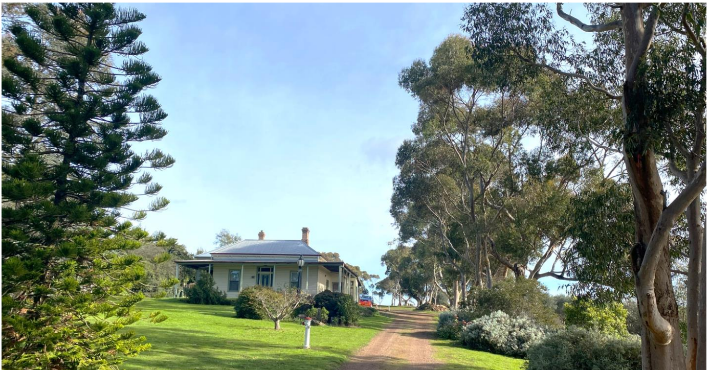
View of 'Avonlea' showing elevated site and Sugar Gums along the north side driveway entry. Source: David Scott, City of Greater Geelong. 2022
