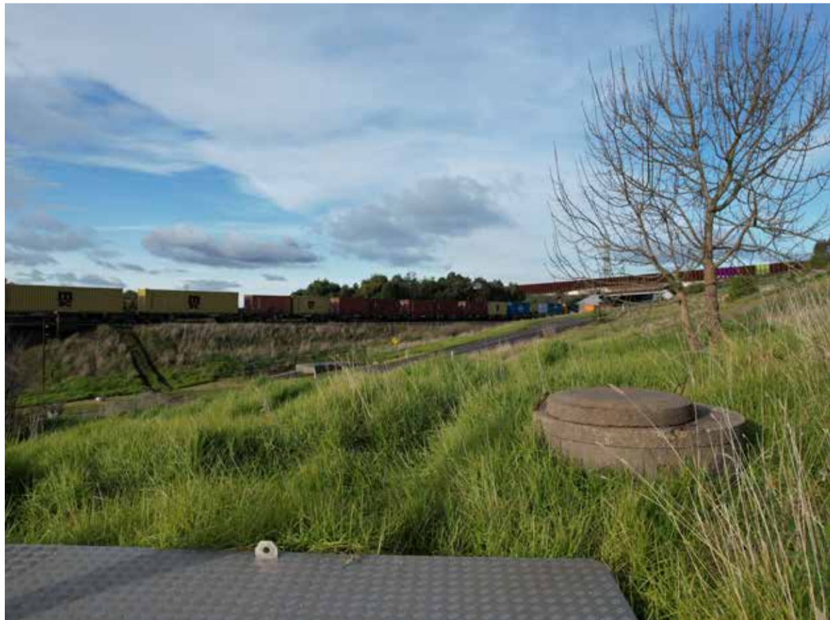
View of rail line looking east
