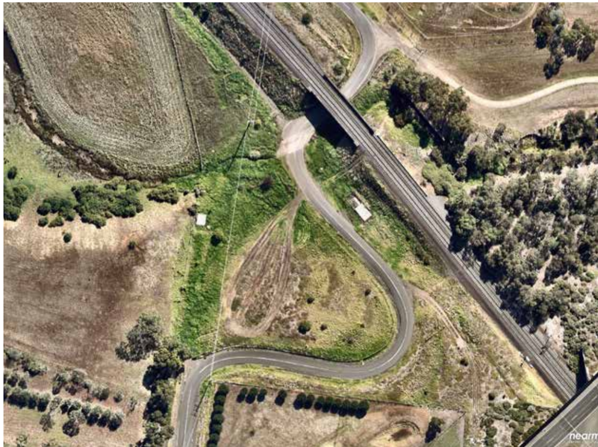
Evidence of 4 x 4 illegal access at Bluestone Bridge Rd
