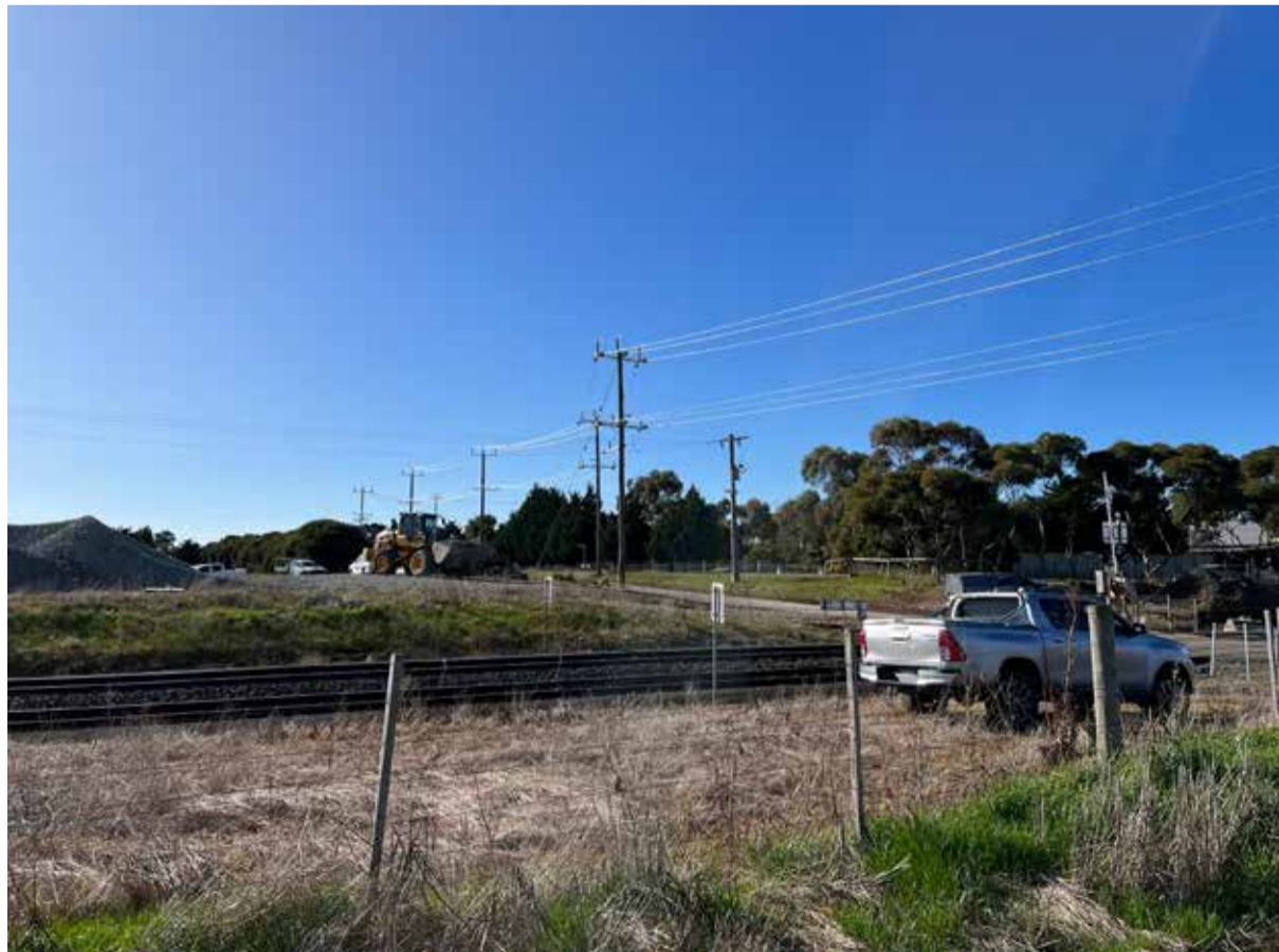
View north along Evans Rd with Ballarat Geelong rail line intersection
