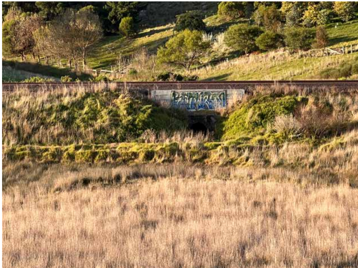
Culvert beneath the Geelong-Ballarat Rail Line
