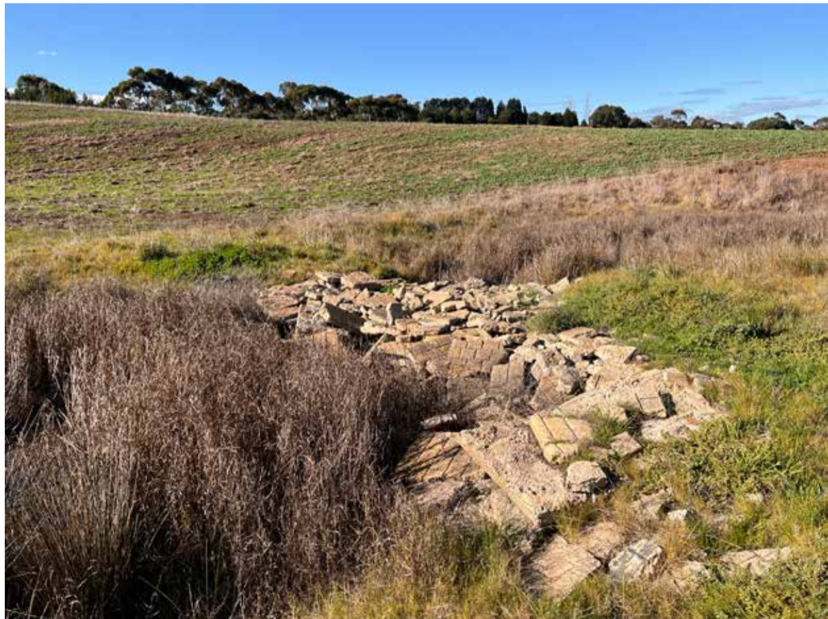
Informal crossing over creek enabling artificial pooling upstream
