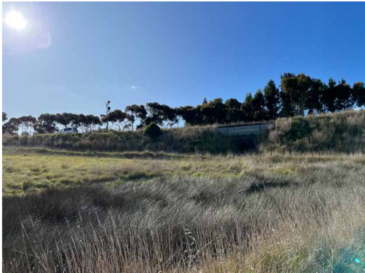
View of culvert beneath Ballarat Geelong rail line
