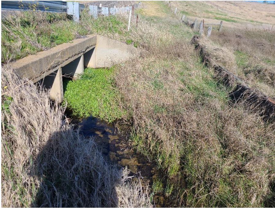
Photo 11 Existing underpass of Cowies Creek at Evans Road. Looking approximately south
