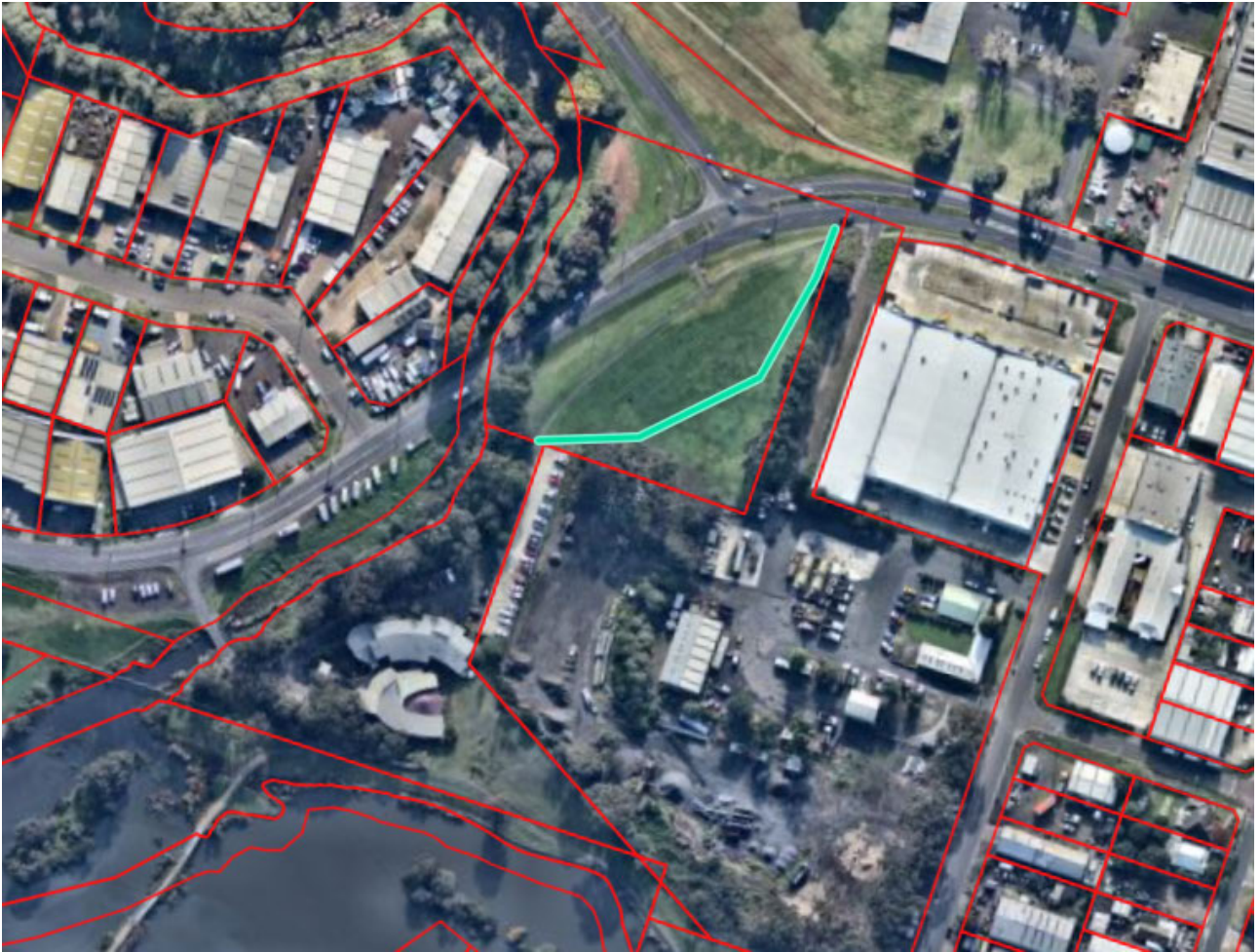
Figure 2. Emergency access through Council land to north
