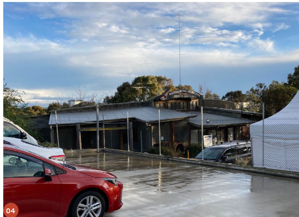
04 Upper secure carpark and health building entry
