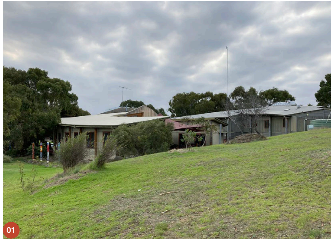
01 Existing buildings - view looking west
