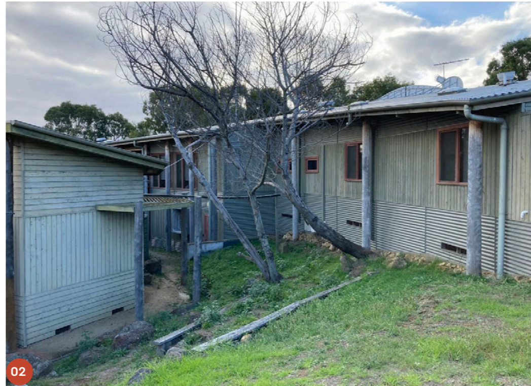
02 South facade of healthcare building
