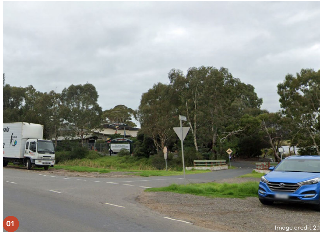
01 Existing entry bridge
