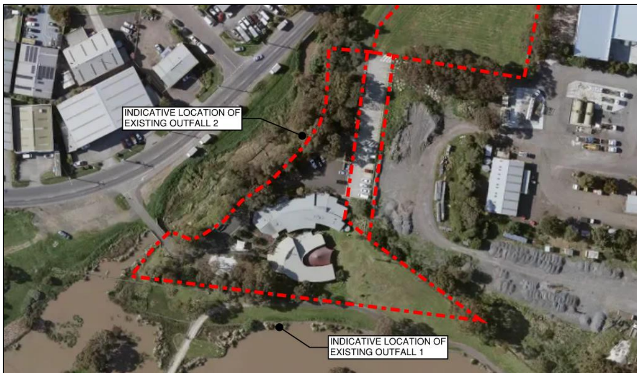
Figure 3 Location of existing outfalls on aerial photography
