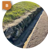
B Beach access gravel path with retaining wall and spoon drain
