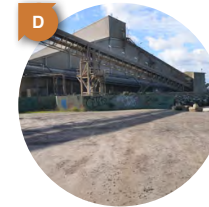
Carpark area and access to neighboring industry. No designated pedestrian area. No existing lighting or surveillance
