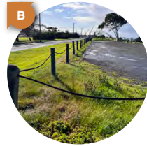
Existing carpark and fencing adjacent to path
