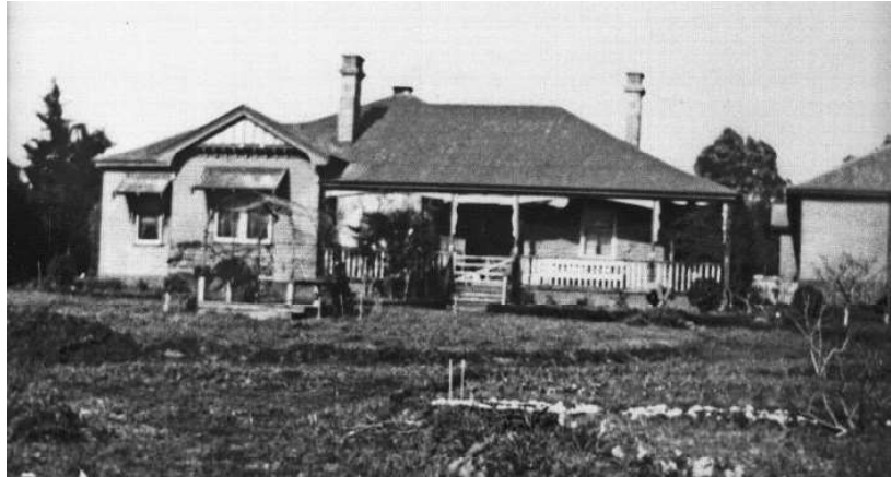
Figure 15: Manager's Cottage with student accommodation adjoining, ND. Source: Ian Wynd Collection. Courtesy of David Rowe.
