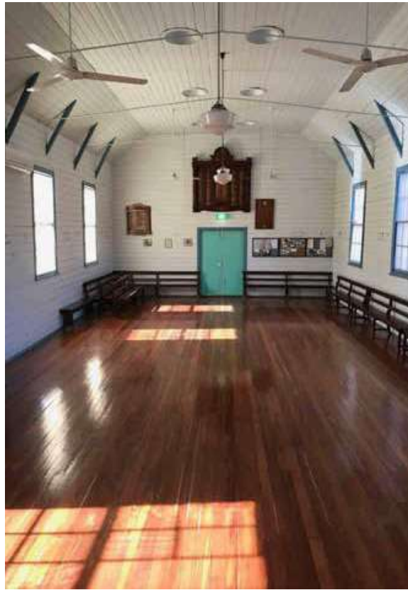
Figure 6: Interior showing timber board linings, timber mansard ceiling and Honour Rolls. Source: Wauru Ponds Hall Facebook
