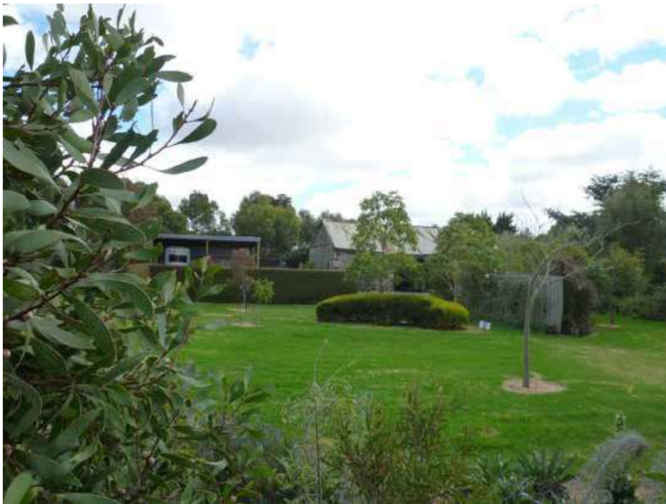
Figure 3: East elevation showing the outbuilding within contemporary landscape setting. Source: David Scott, City of Greater Geelong, 2022
