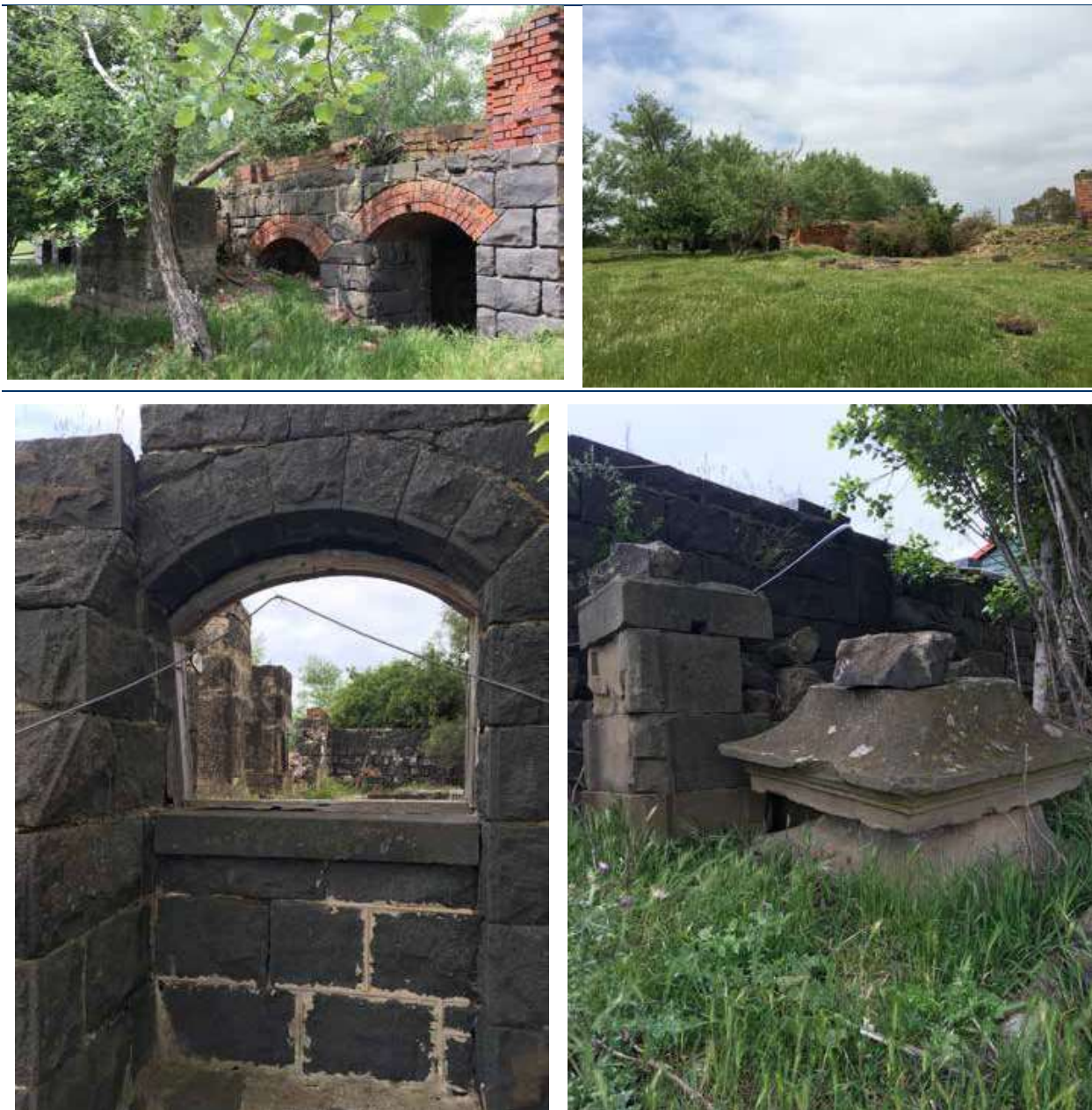
Figure 6-10: Remnant bluestone ashlar walls with segmentally arched window and architectural remains. Source: Jennifer Bantow, 2020
