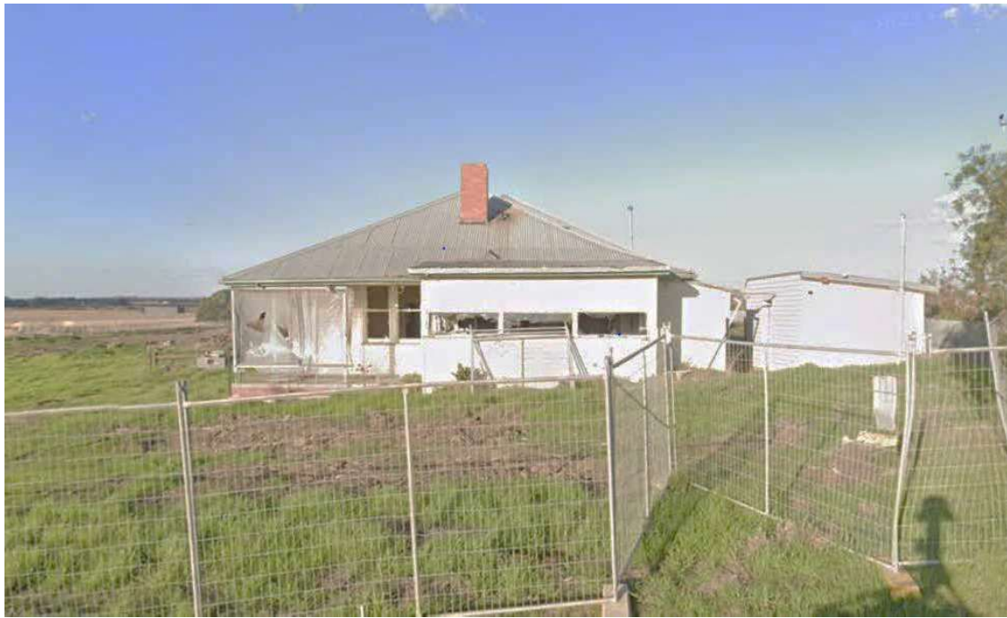
Figure 6: Manager's Cottage(former) showing skillion addition (west elevation) Source: Google Streetview, May 2023
