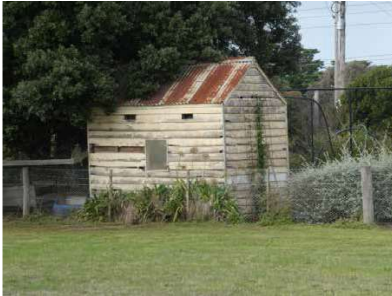
Figure 6: Early-mid C20th Garden shed situated north of homestead. Source: David Scott, City of Greater Geelong, 2022
