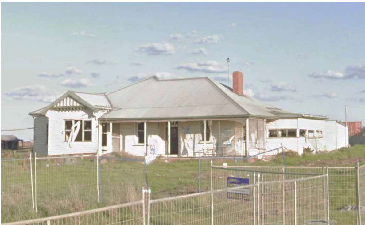
Figure 5: Manager's Cottage (former) showing hipped roof forms, gable, and brick chimney (north elevation) Source: Google Streetview, May 2023
