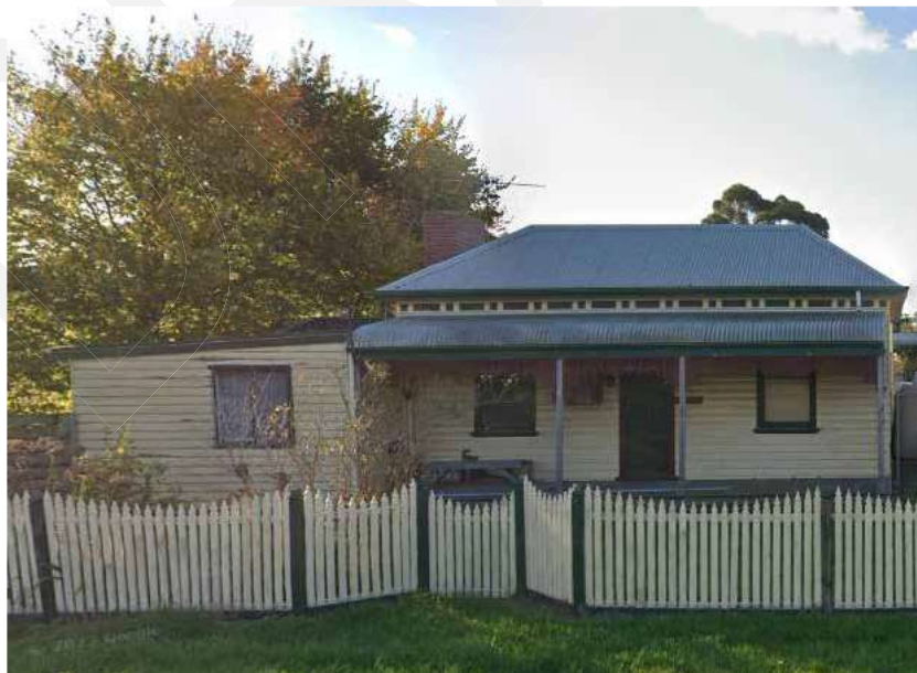
Figure 4: 'Iolanthe', showing 20 th century addition (south elevation). Source: Google Street View, January 2024
