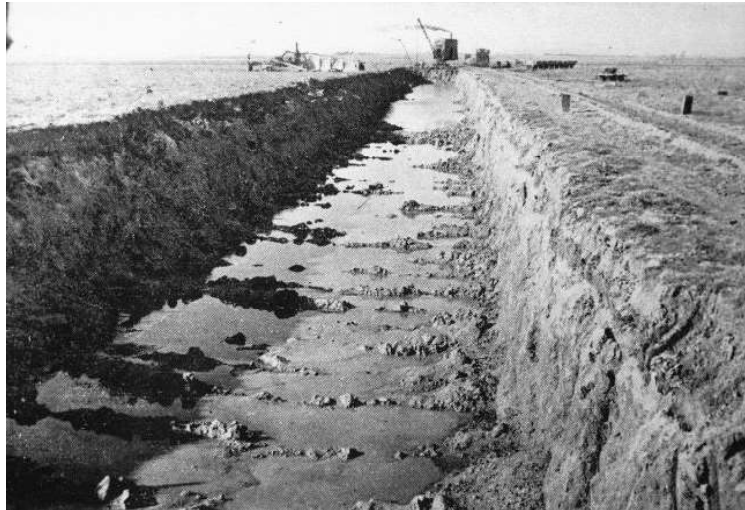
Figure 18: Excavation of Barwon Channel to generate a navigable shortcut and fill for the levee bank, Sparrovale, c.1912. Source: Ian Wynd Collection. Courtesy of David Rowe
