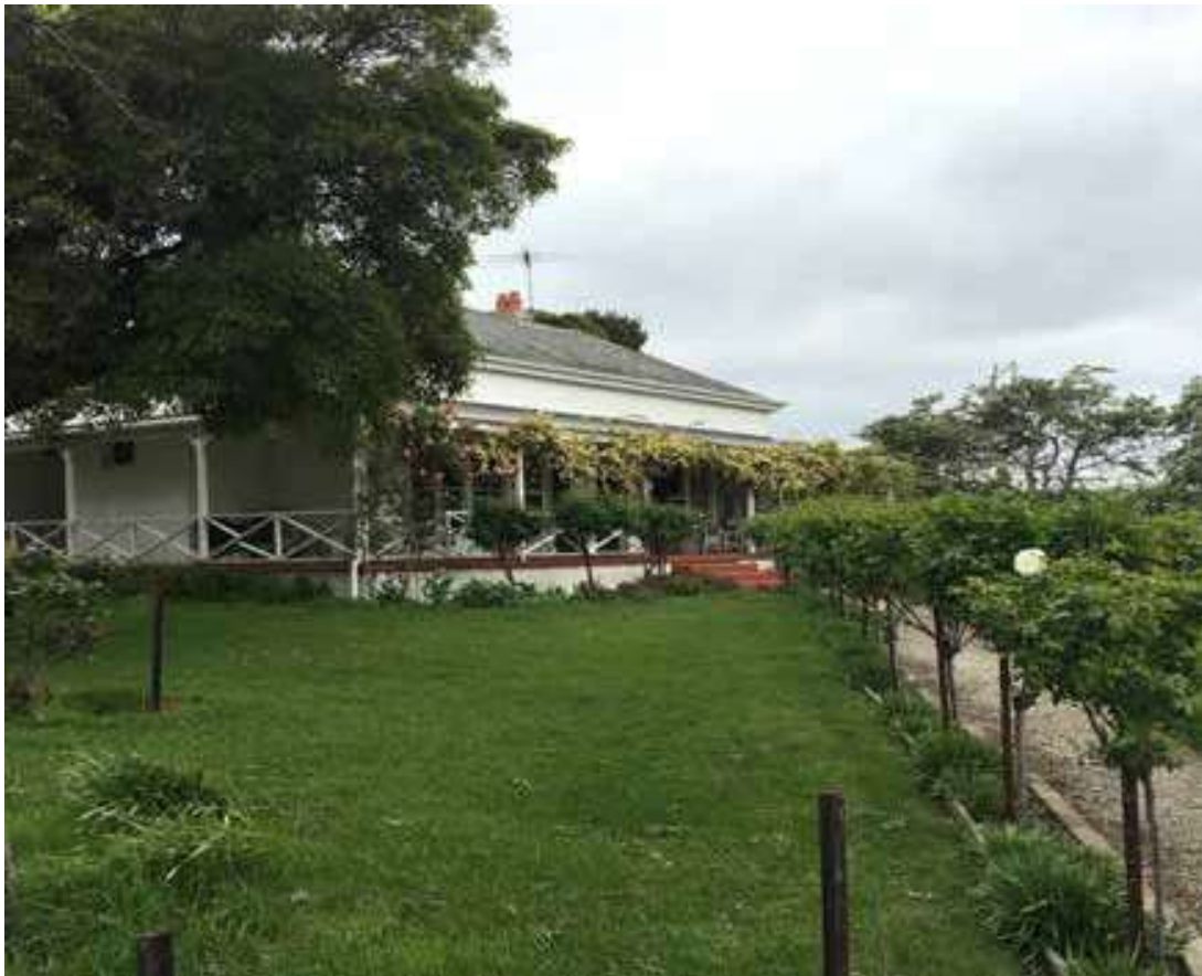
Fig 13. North elevation showing replacement c1990s wrap-around verandah, new chimney pots and garden plantings. Source: Jennifer Bantow, 2020.
