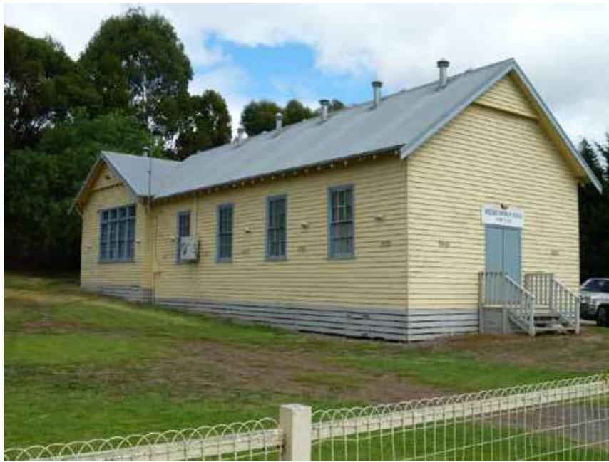
Figure 4: North elevation showing details of the Waurn Ponds School addition. Source: David Scott, City of Greater Geelong, 2022
