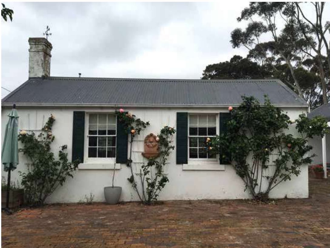
Figure 14: Outbuilding attached to residence (early kitchen or washhouse), north elevation showing early-design 6-pane window sashes and 1990s shutters and modern roofing. Source: Jennifer Bantow, 2020
