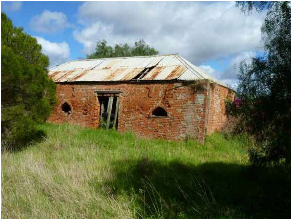
Figure 3: Stables, east elevation showing hipped roof, structural iron S-ties and pointed arch openings. Source: David Scott, City of Greater Geelong, 2022.
