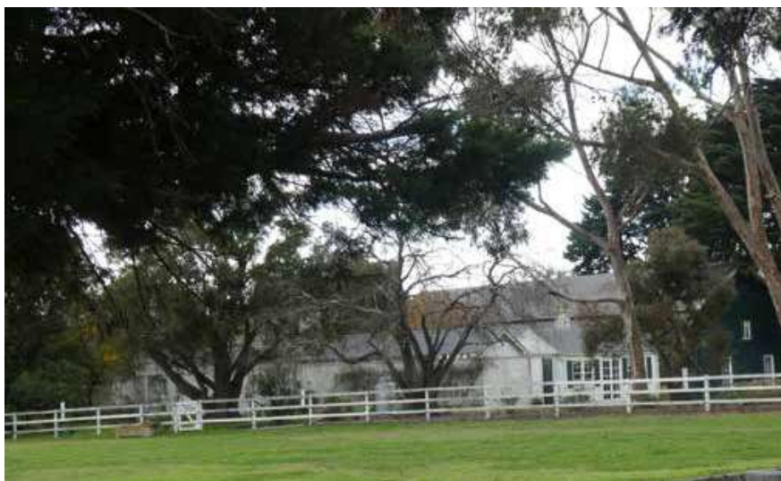
Figure 12. ‘Greenbank’, west elevation (LH) David Scott, City of Greater Geelong, 2022
