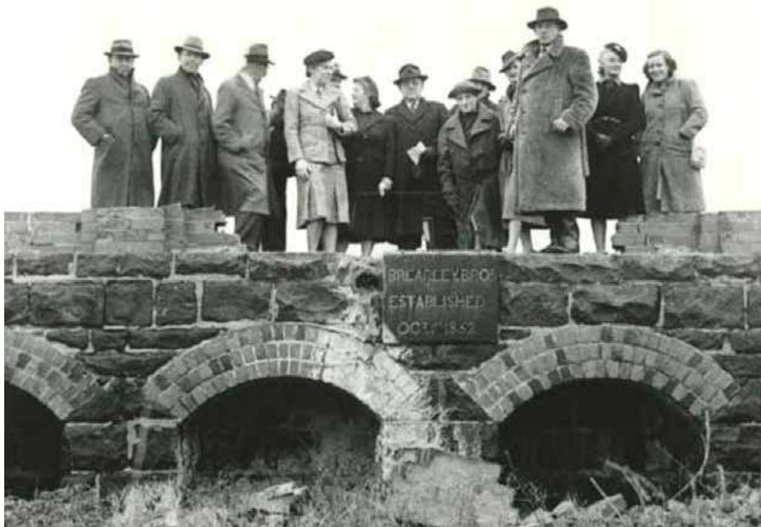
Figure 18: Geelong Historical Society Members at Brearley's Tannery, c.1950. Original foundation stone, removed c1990 Source: Geelong Heritage Centre
