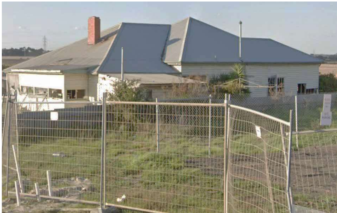
Figure 7: Manager's Cottage (former) showing hipped roof forms and skillion addition (south elevation) Source: Google Streetview, May 2023
