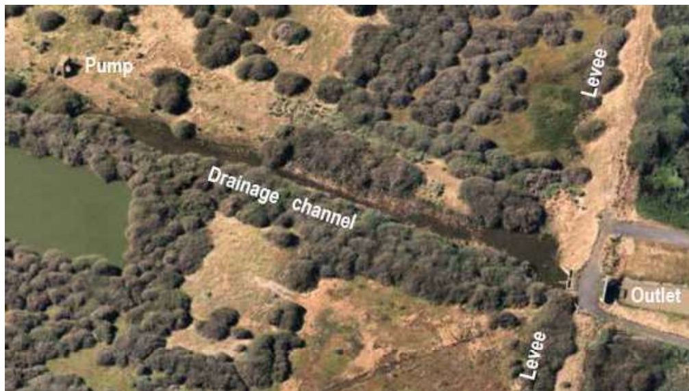
Figure 8: Intersection of drain with levee bank, and site of early windmill. Source: Nearmap 2019
