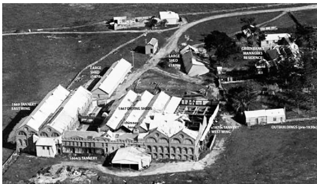
Figure 5: Aerial view from north/river showing building sites labelled as per Features Plan. Charles Pratt 1930. Source: State Library of Victoria
