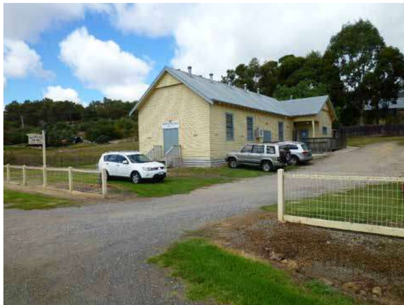
Figure 5: West elevation showing details of the Waurn Ponds School addition. Source: David Scott, City of Greater Geelong, 2022
