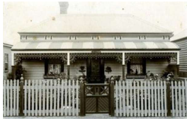
Figure 67 Victorian dwelling with pointed timber picket fence, expressed posts with decorative cappings and timber gate. Source: Emerald Museum.
