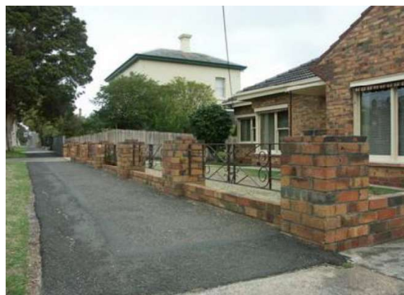
Figure 85 Low solid brick fence with open bays with trussed geometric panels.
