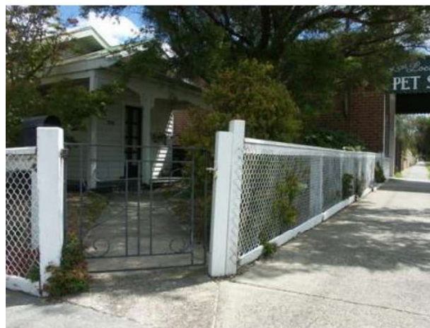
Figure 82 Interwar bungalow styled dwelling with a capped timber post and chain mesh front fence having open geometric steel gate.
