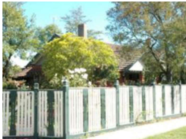
Figure 80 Capped timber picket fence to an interwar bungalow styled dwelling.
