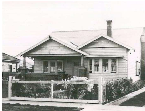
Figure 81 Timber post and rail, and woven wire fence to an interwar bungalow styled dwelling.
