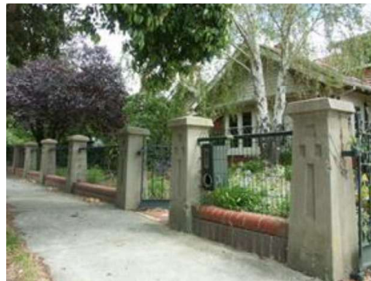
Figure 78 More substantial woven wire fence to large property with rendered piers and brick plinths.
