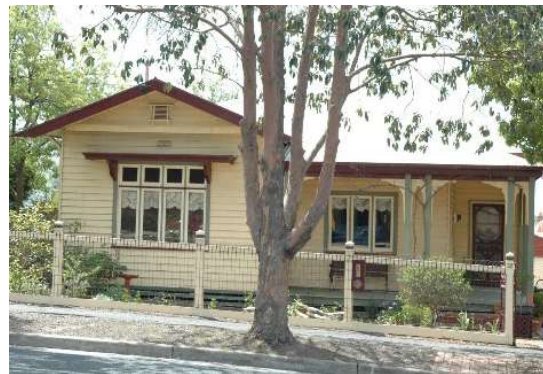
Figure 89 Fence following gradient of boundary slope.
