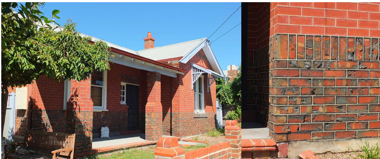
Figure 11 Bungalow, Newtown, 1920s . Bungalow featuring distinctive brickwork construction enhanced by tuckpointing repairs.
