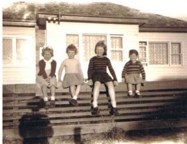
Figure 86 Horizontal timber paling fence to postwar bungalow. Source: Lorraine Huddle.
