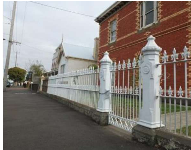
Figure 70 Substantial late Victorian brick dwelling with iron palisade fence having cast iron piers and bluestone plinths.
