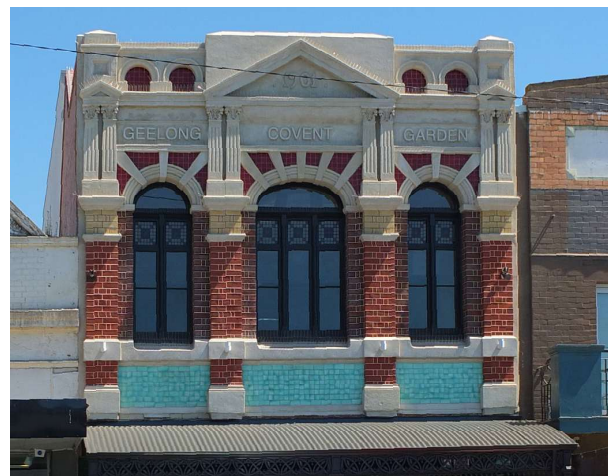
Figure 35 Geelong Covent Garden, Moorabool Street, Geelong, showing the exterior as largely originally intended. The overpainting was removed by approved poultice method, leaving the surface of the brickwork and tiles undamaged.
