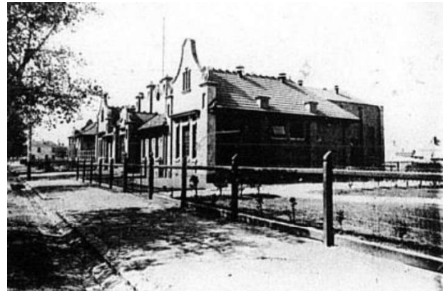
Figure 77 Capped timber post and woven wire fence. Source: News of the Week, 1916.
