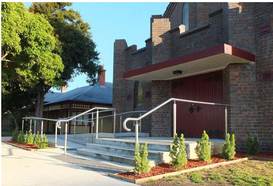
Figure 46 Former Shenton Methodist Church (now part of Geelong High School), Geelong. New ramp and stairs added for accessibility.
