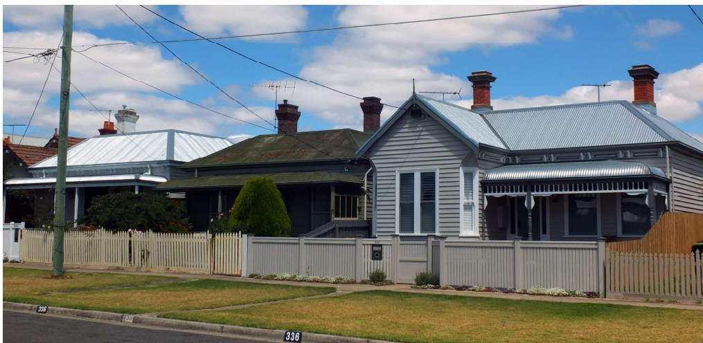
Figure 36 Streetscape, East Geelong. A Victorian dwelling (left) with a new Zinalume® roof and a Late Victorian dwelling (right) with a new galvanised steel roof.
