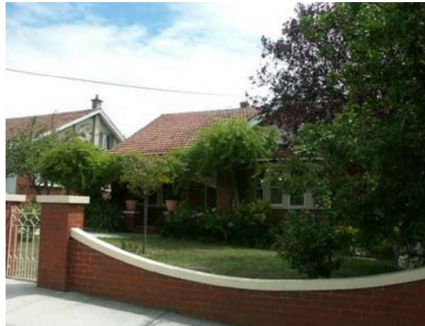
Figure 83 Interwar solid brick fence, being sufficiently low not to obstruct the view to the front garden.
