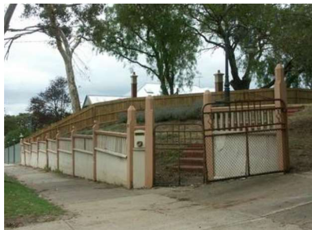
Figure 76 Detail of Federation era ripple iron and timber fretwork fence, with scrolled metal and wire vehicular and pedestrian gates.
