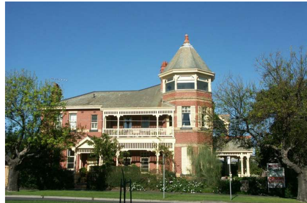
Figure 59 Pevensy House, Geelong.
